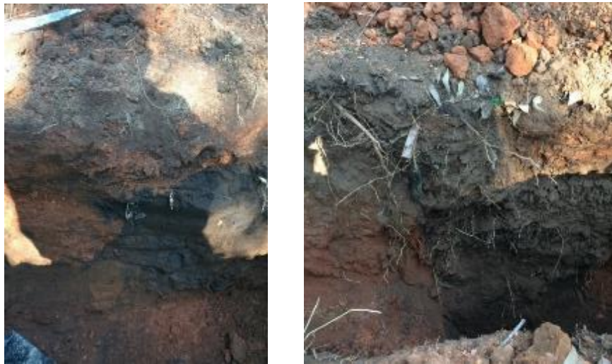
Figure 6-9: Observed visual differences in surrounding soil and buried sludge trenches, demonstrating a continued difference after >10 years
