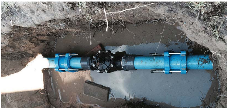
Image of an installed AquaTrip (Credit: Splash Plumbing)
