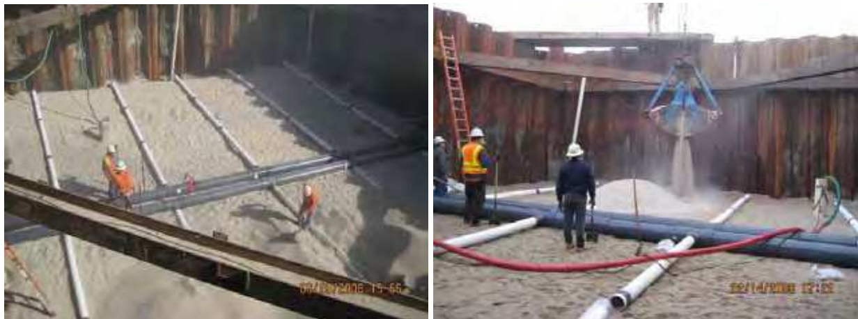
Figure 9.1 Under-ocean floor seawater intake and discharge demonstration system
