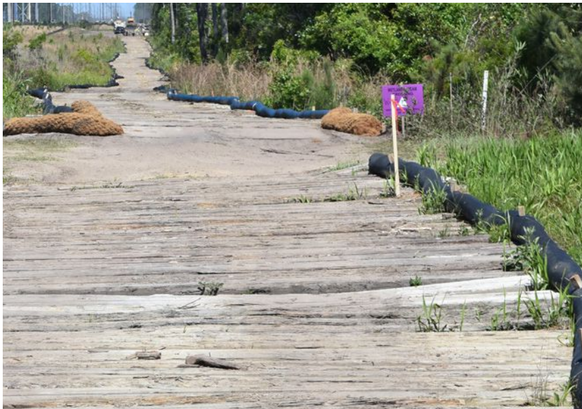
Proper signage at areas such as this wetland crossing can improve awareness and assist with permit special provision compliance.
