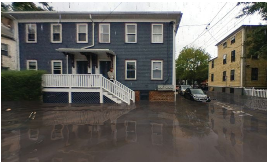
Climate change will exacerbate the frequency and severity of storms, which results in flooding from stormwater and sewer overflows.
