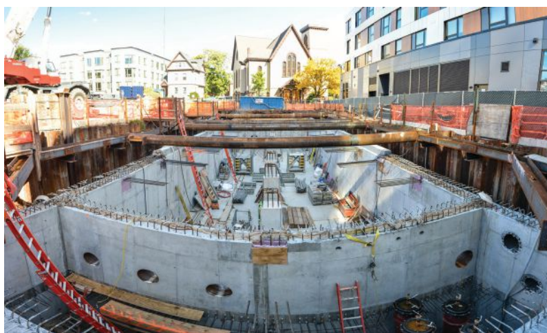
The stormwater tank under construction in Fall 2019. The simultaneous construction of the Market Central towers (building shown on the right), less than 8 feet from the tank, required extensive coordination and geotechnical monitoring.
