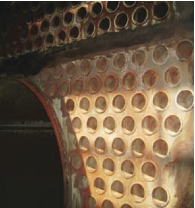
Orange/reddish color in the tube sheet of a firetube boiler suggests some corrosion has occurred in the fireside. Cortec® image.
