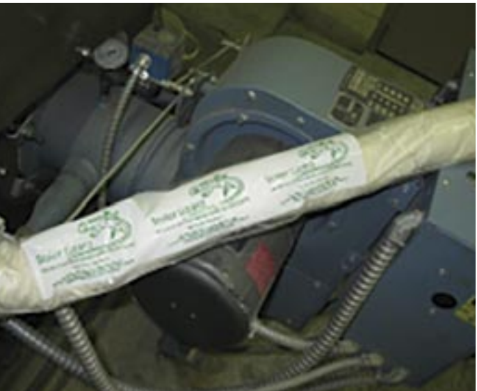
A classic example of VCI dry layup: VCI powders packaged in a water-soluble tube that dissolves when the boiler is refilled. Cortec® image.
