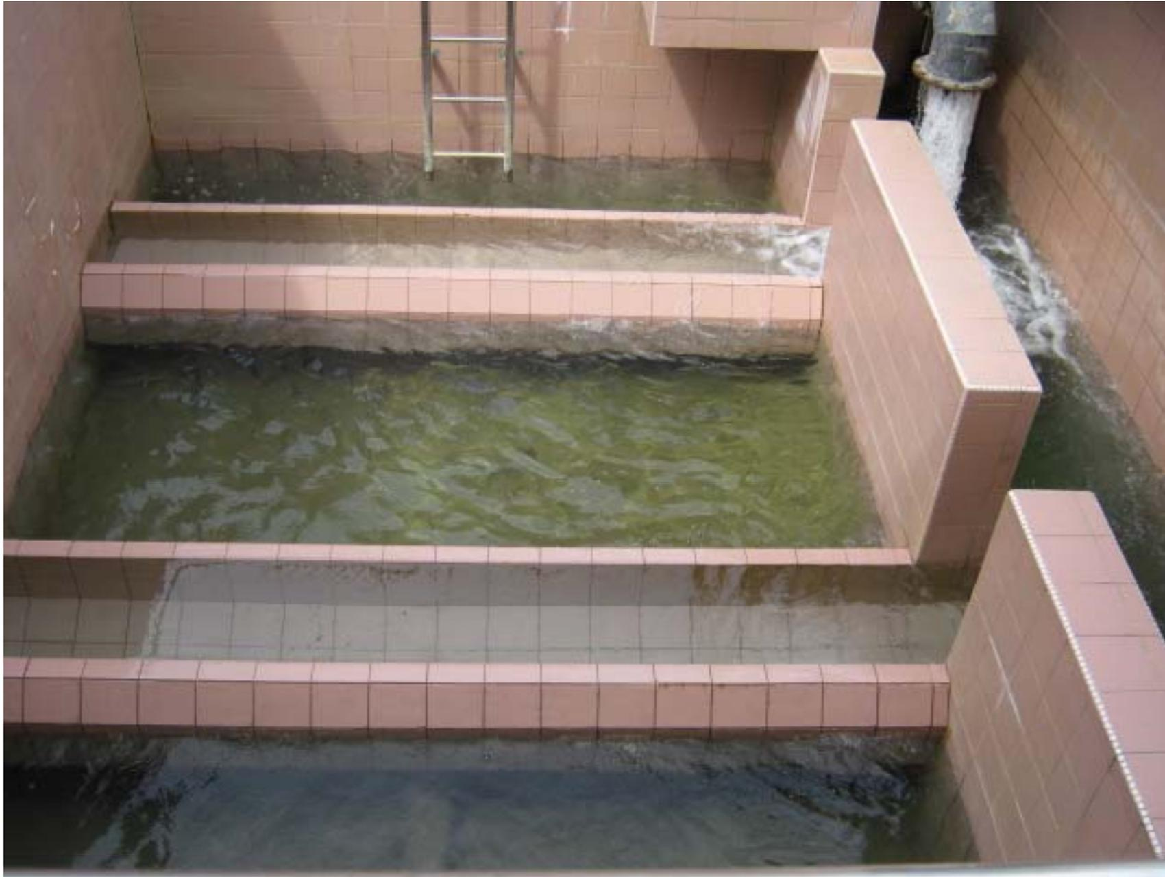
**Figure 5.12 : Rapid sand filter during filtration**
