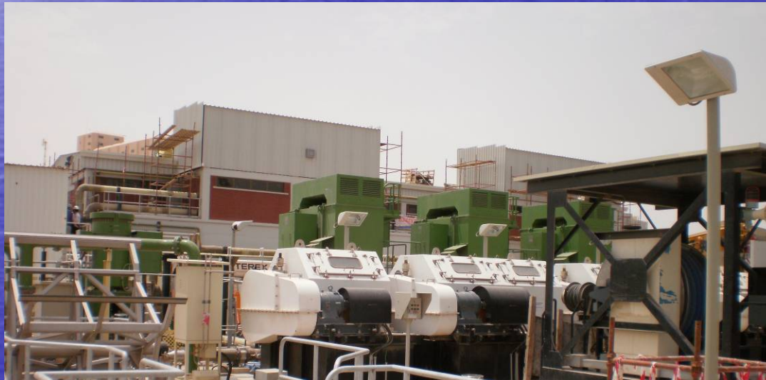
Plant Intake/Screening Structure in Foreground, Clari-DAF Building in Background
