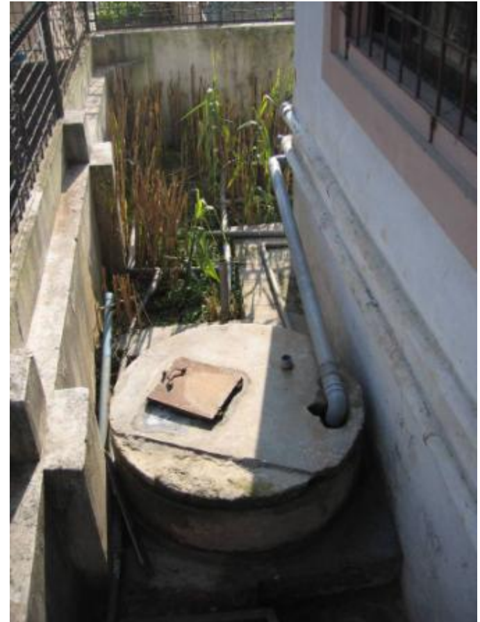
Dug well for groundwater collection and recharge
