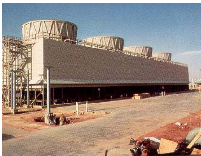
Figure 4-9. Counter-Flow Cooling Tower
