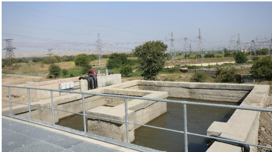
*Figure 26 - Inlet chamber with large traps (Image taken by author)*
