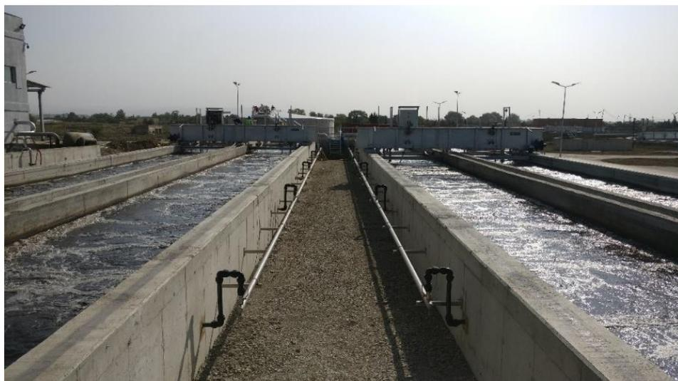
Figure 28 - Grit and Grease Chambers. Compressed air pipes are visible on the side of the chambers (Image taken by author)
