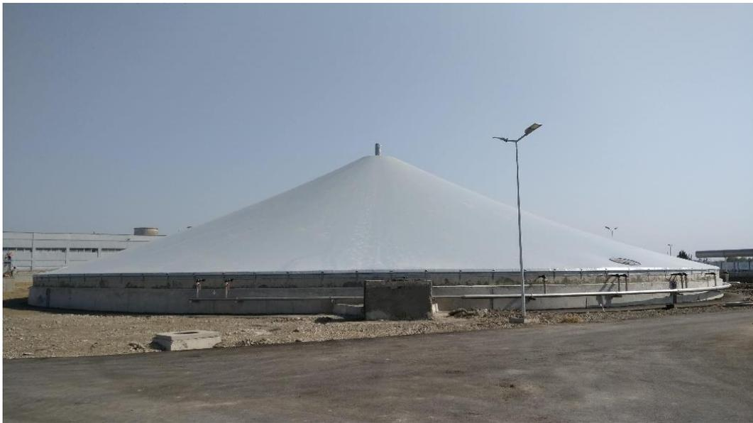
*Figure 32 - Sludge Stabilization Tank (Image taken by author)*
