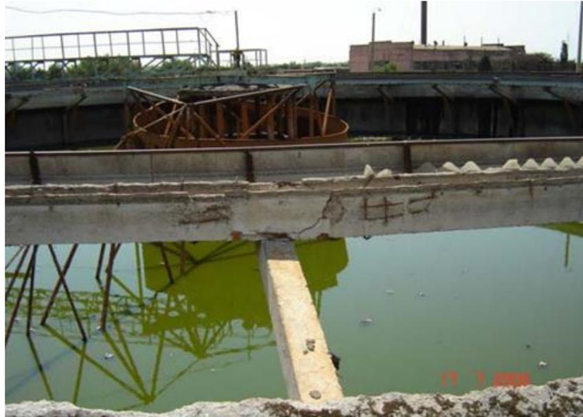
*Figure 30 - Primary clarifier before rehabilitation. Source - (Shubitidze, 2006)*
