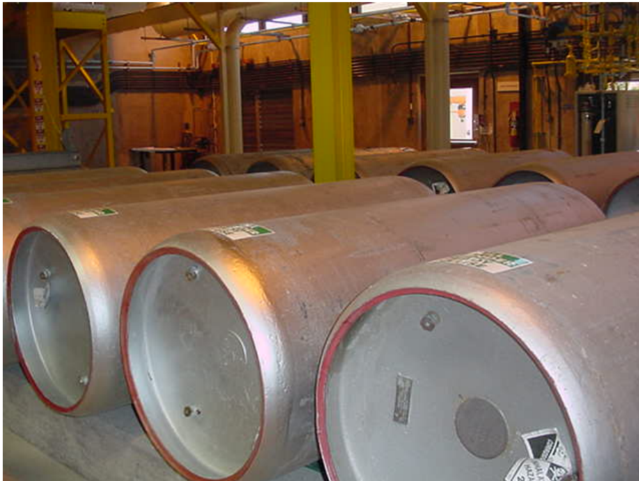
1-ton chlorine containers, rear side of container.
