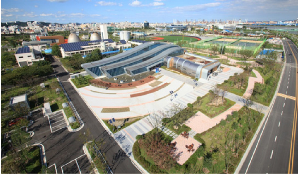
Figure 28 | Panoramic view of Wastewater Reuse Facilities in Pohang
