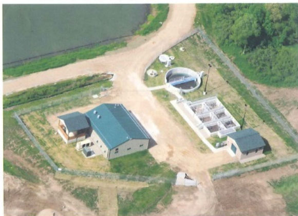
Upgraded Bloomingdale WWTP is Simple & Robust
