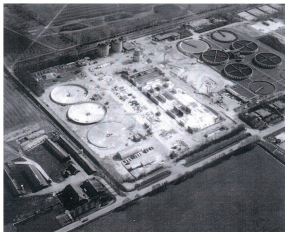
Figure 1.8 – Overview of a WWTP (under construction)
