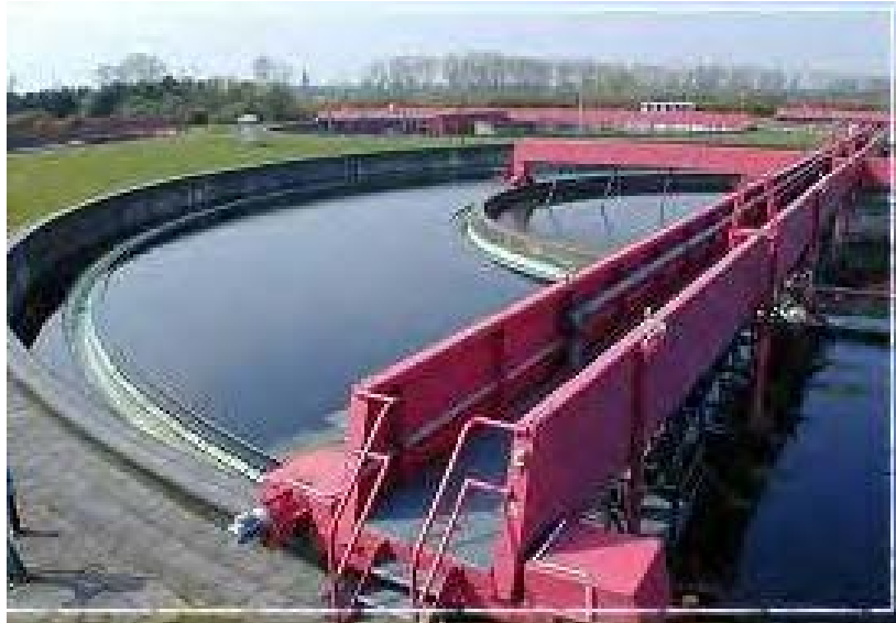
Round shaped tank with scraper bridge Rectangular tank with lifted scraper shield
