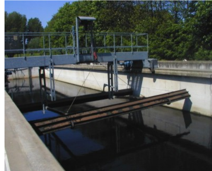
Round shaped tank with scraper bridge Rectangular tank with lifted scraper shield
