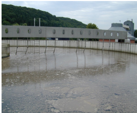
Overfall weir with submerged wall
