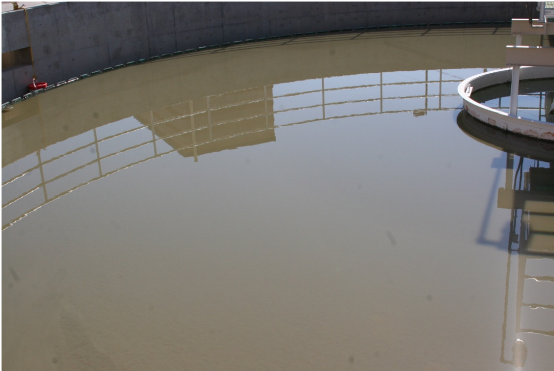
Top- Pre-sedimentation basin
