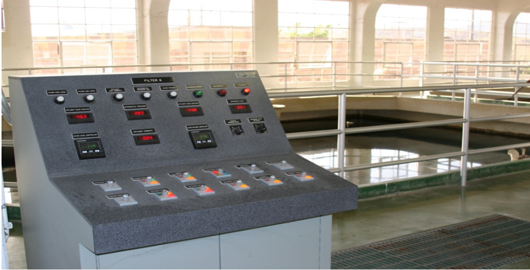
This is a water treatment filter control panel.
