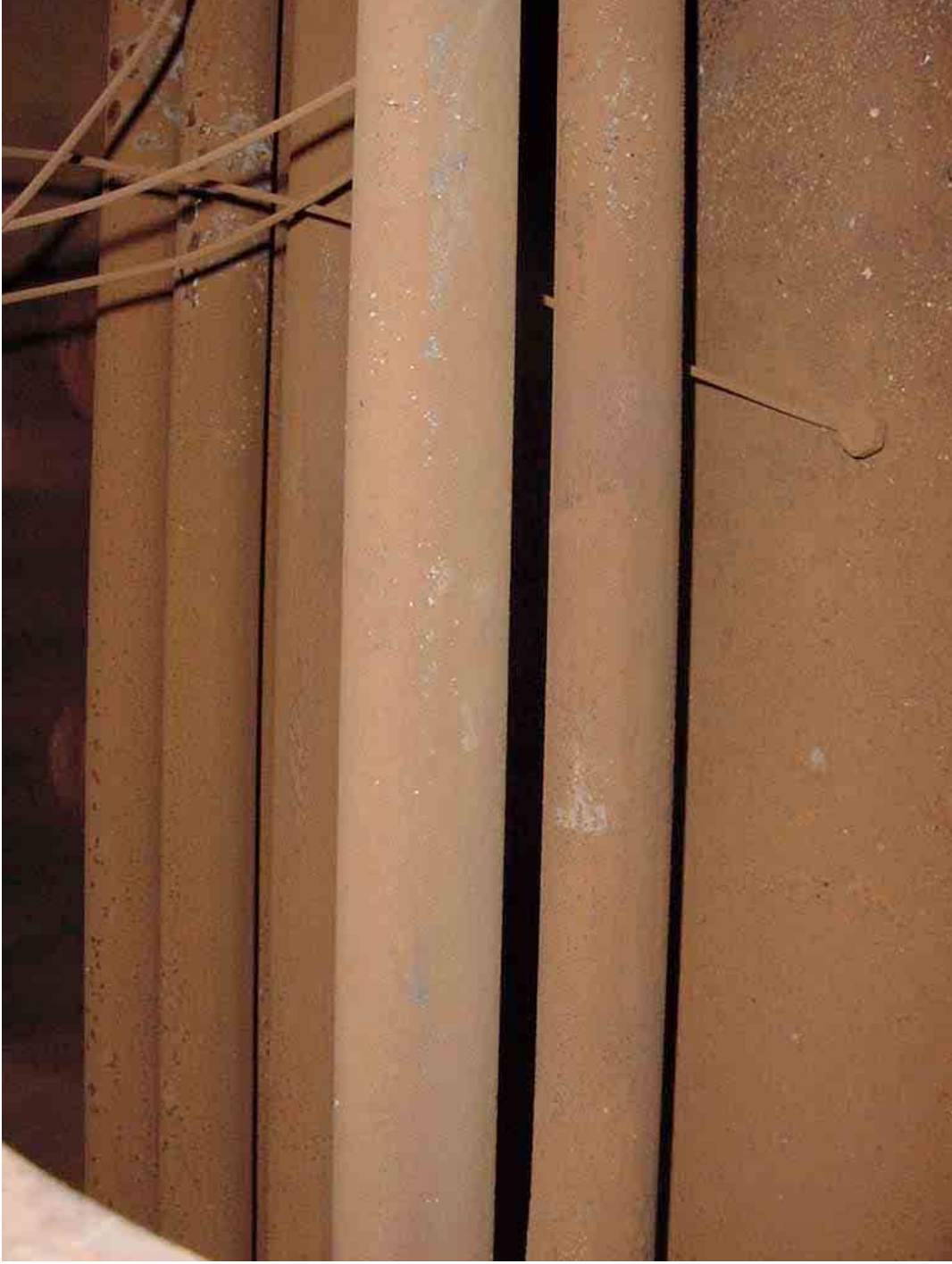
Figure 18 Smoke tubes after repeat runs with no treatment
