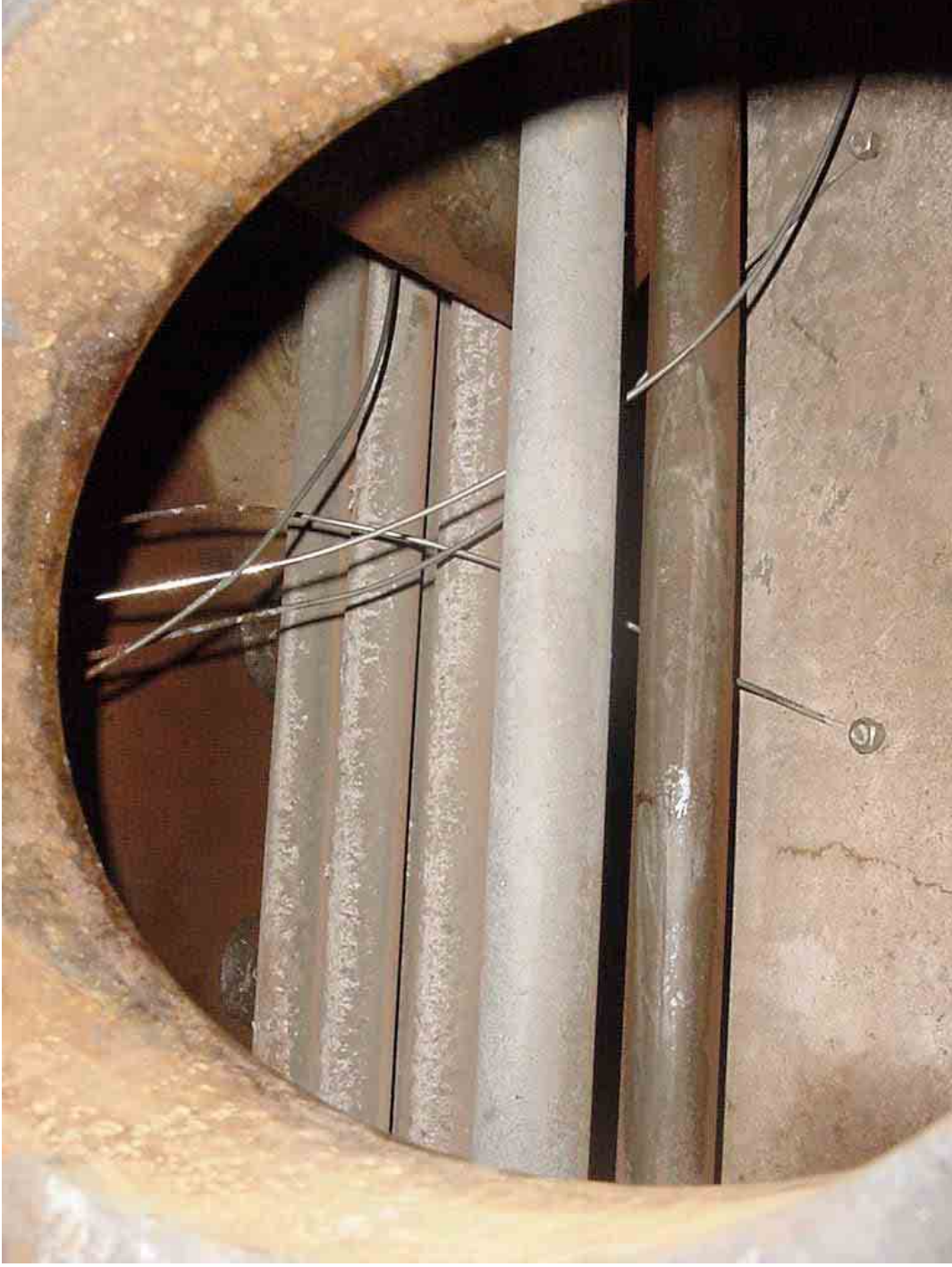
Figure 17 Smoke tubes before repeat runs with no treatment
