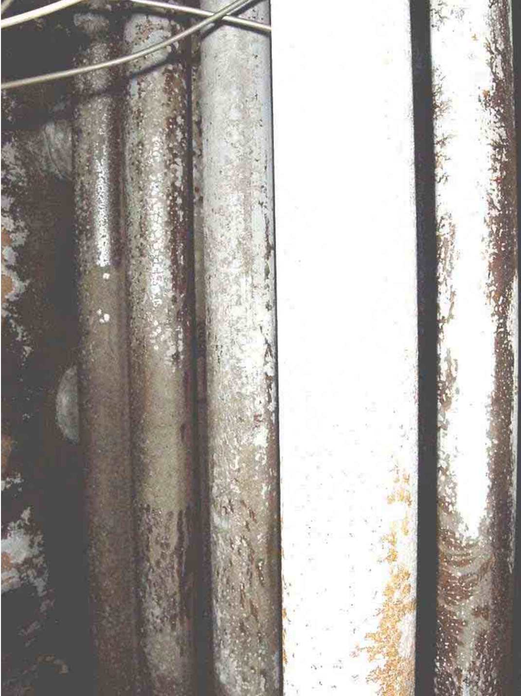
Figure 19 Smoke tubes before tests with Device B
