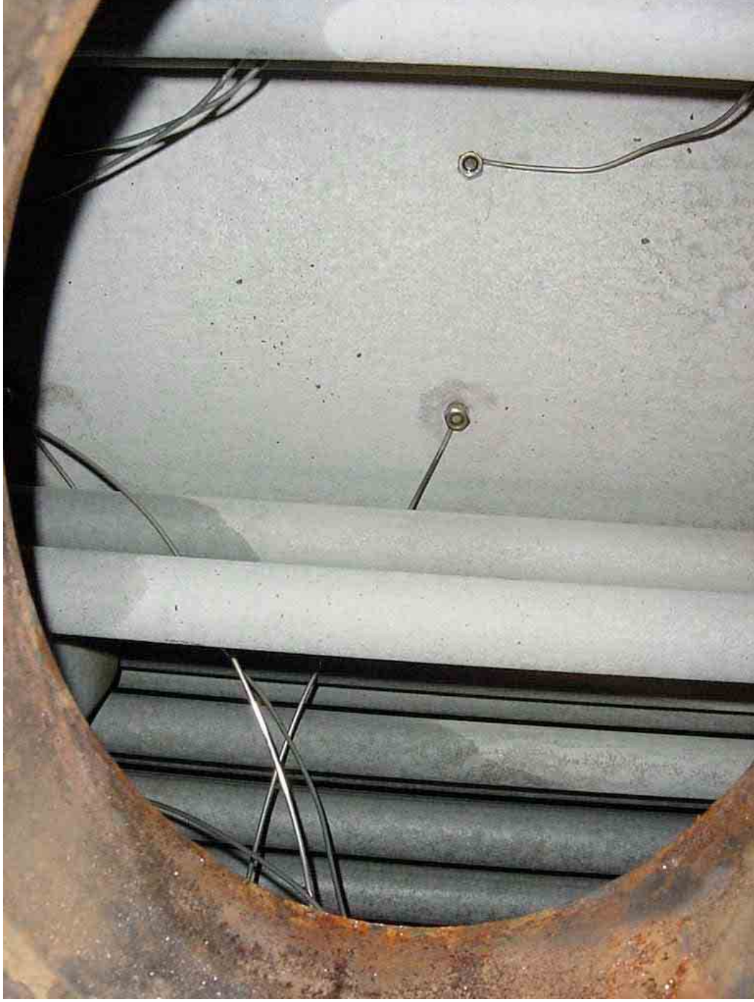
Figure 32 Cleaned boiler surfaces prior to repeat tests on Device A
