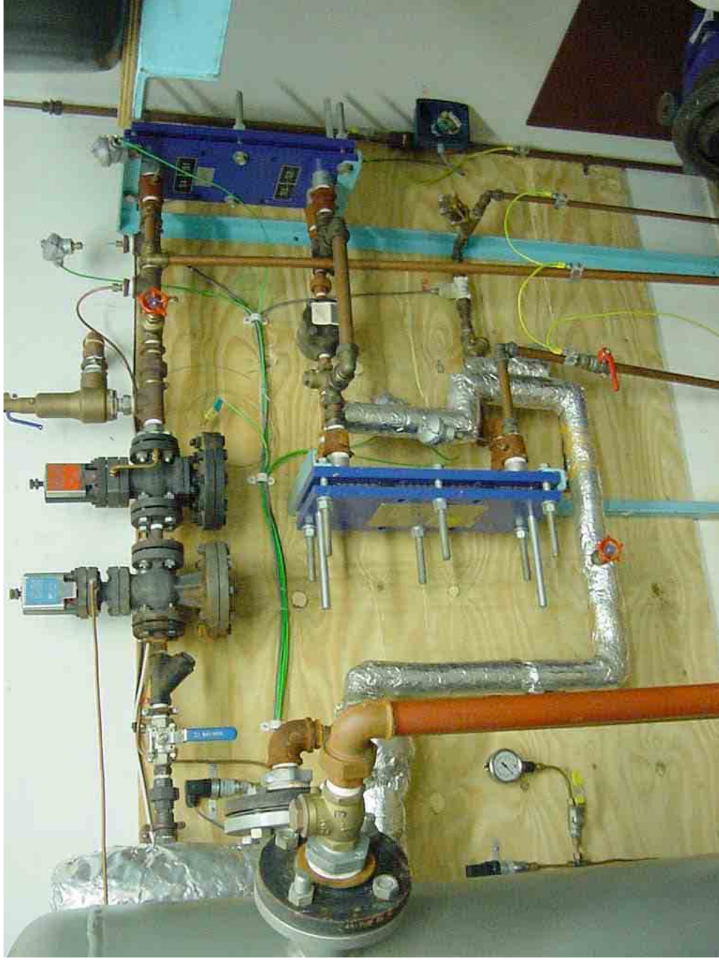
Figure 3 Steam control circuit components
