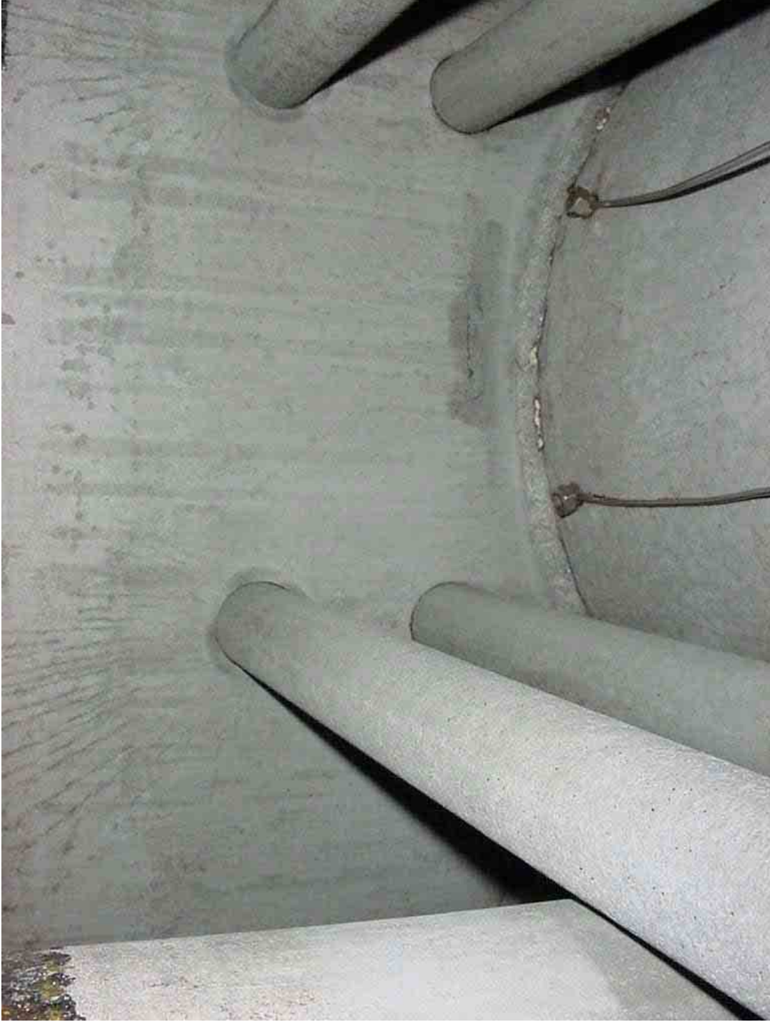
Figure 33 Cleaned boiler surfaces prior to repeat tests on Device A
