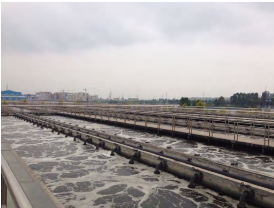
Figure 30: Aeration tank in a textile effluent treatment plant in China
