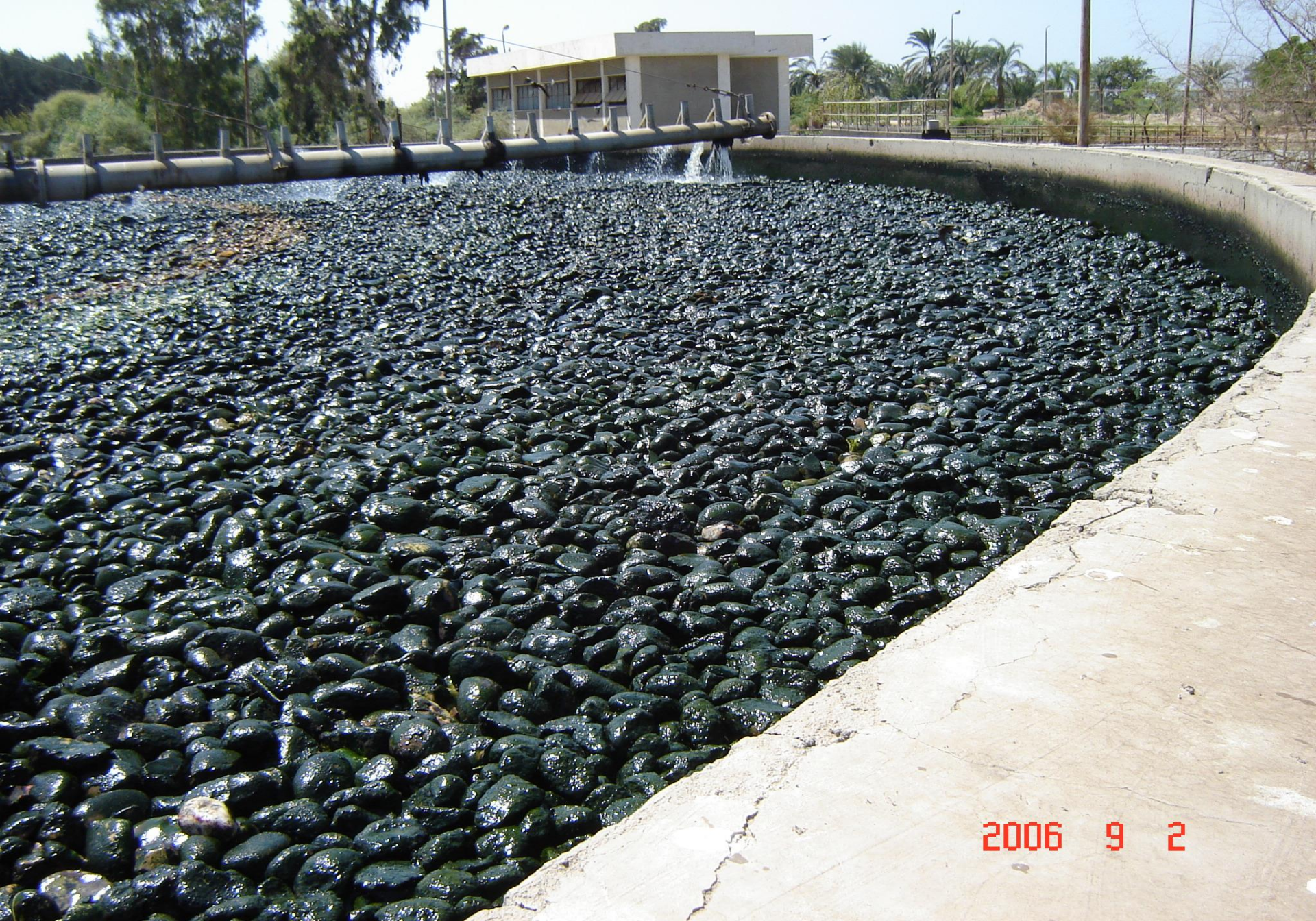
Trickling Filter
