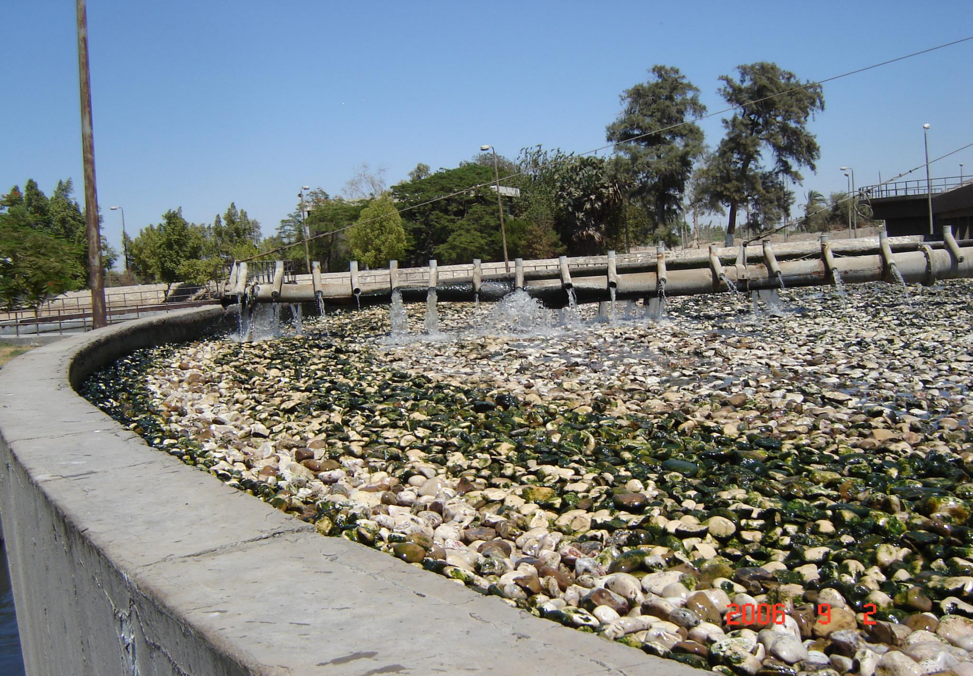
Trickling Filter
