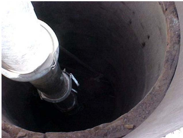
Looking down inside the manhole.
