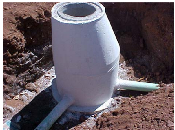
Newly finished Manhole and Laterals.
