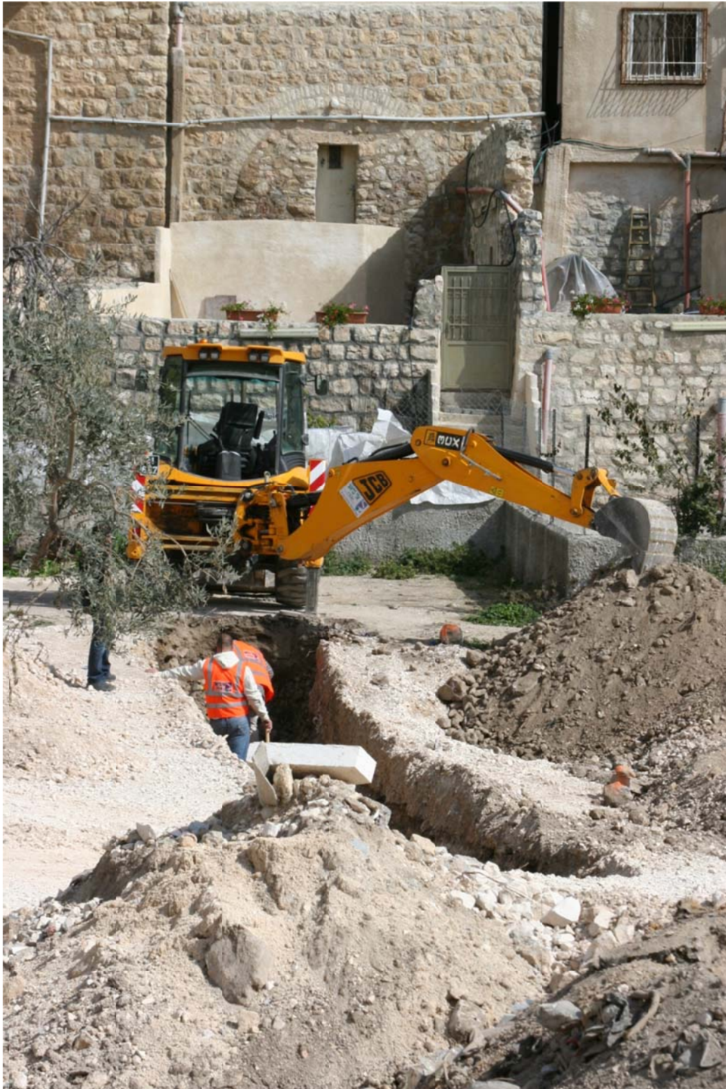
Normal day for a collection system operator. These men dug for several hours to find a broken sewer line. Some days are harder than others.
