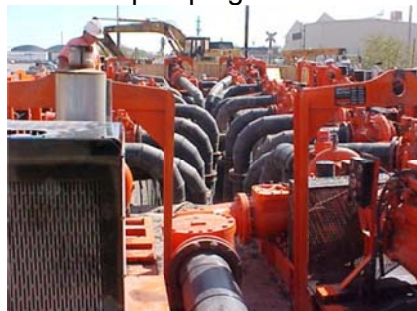
Pumps at a temporary sewer manhole by-pass.
