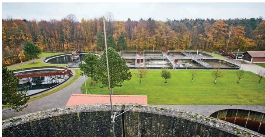
WWTP in the town of Stadtlahn, North Rhine-Westphalia
