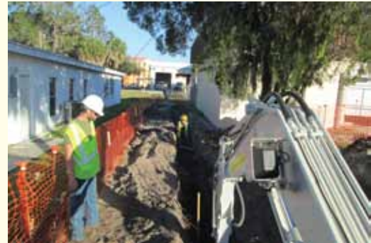
Installing new instrumentation and control systems.
