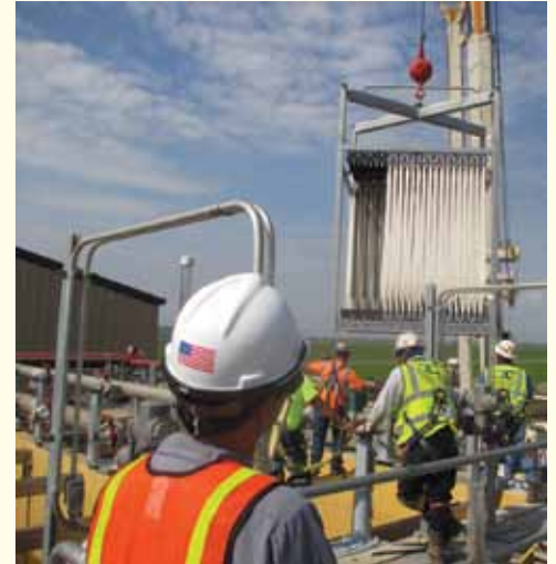
The level of membrane bioreactor water treatment technology used at the BioKyowa facility goes beyond the norm for an industrial discharger.
