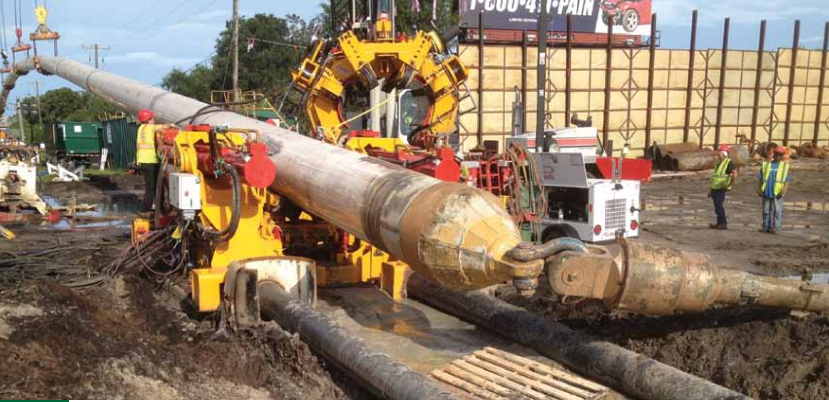
Construction of a new water supply line in Jacksonville, Florida.
