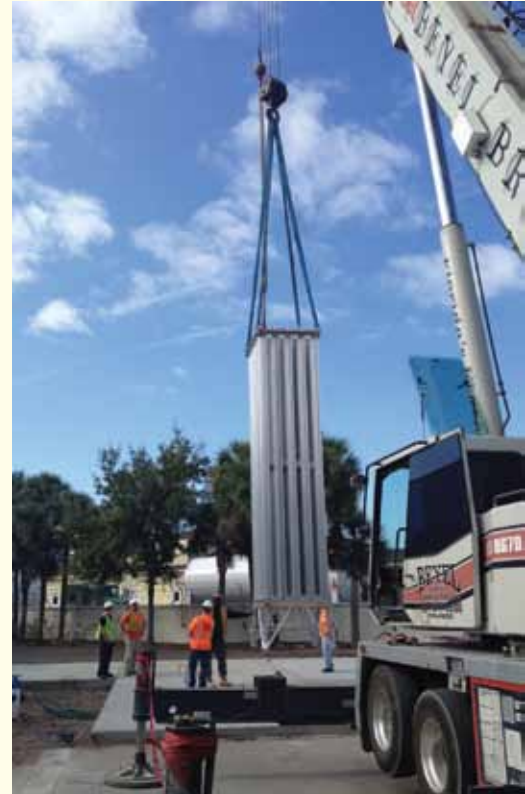
The 14-month construction phase included replacing three ozone-generator systems and installing a new liquid oxygen system, new motor control centers, feed piping, and retrofitting.
