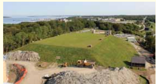
The Lawton Valley water treatment plant site, showing the buried 4-mg reservoir that was demolished to allow the new treatment plant to be built in its place.
