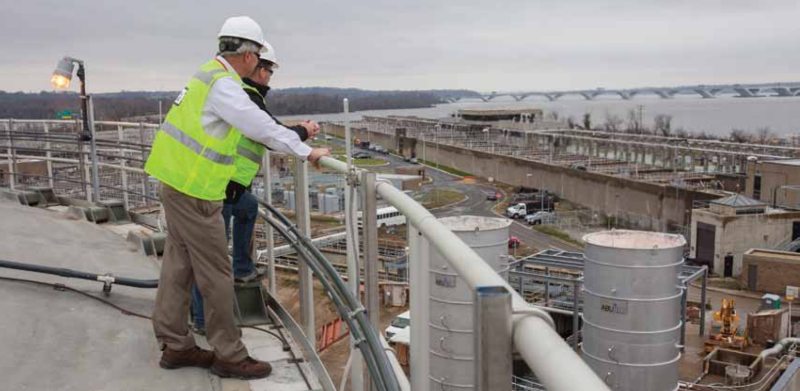
Managers look out over the DC Water (Cambi) Energy Recovery System.
