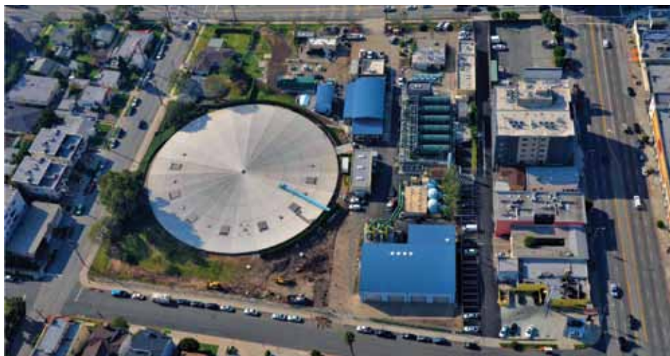
Charnock Well Field Restoration Plant provides quality water to California customers.
