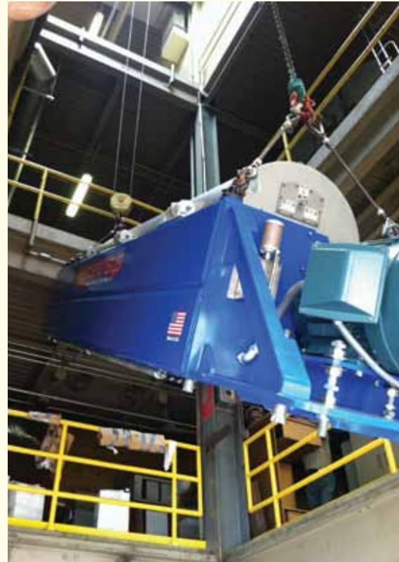
Installation was accomplished with one dewatering train on line at all times.
