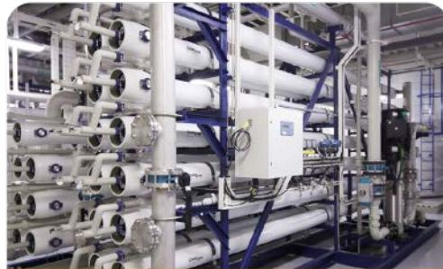
Sadara, Saudi Arabia Seawater Ultrafiltration/Reverse Osmosis 178,000 m 3 /d
