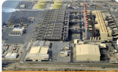
Fujairah, UAE Hybrid Desalination 136,500 m 3 /d
