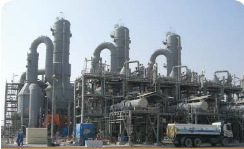
Shell Pearl GTL, Qatar Zero Liquid Discharge HPD® technology
