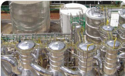
Veracel Celulose, Brazil Black liquor evaporator system HPD® technology
