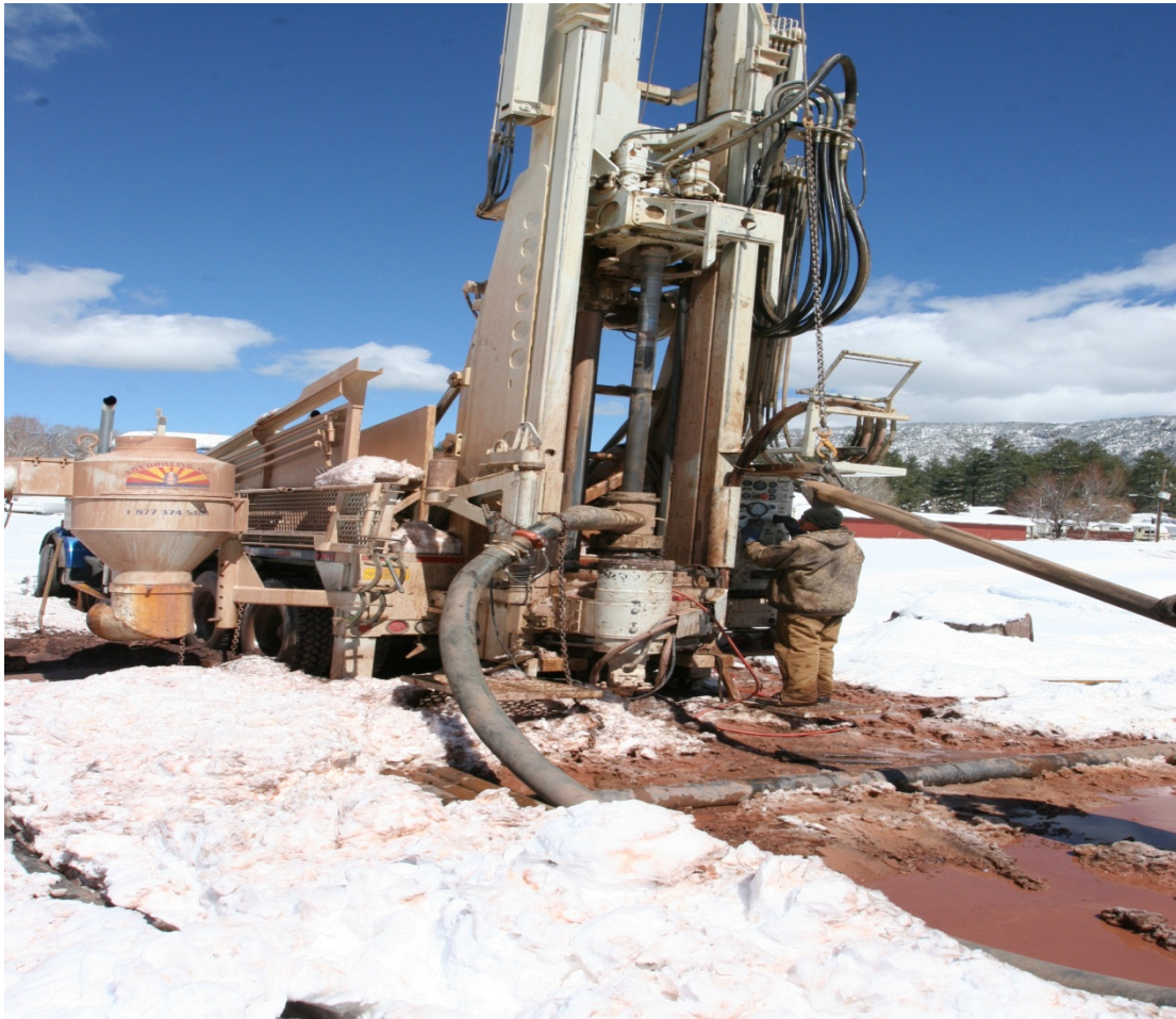
A drill rig in the snow.
