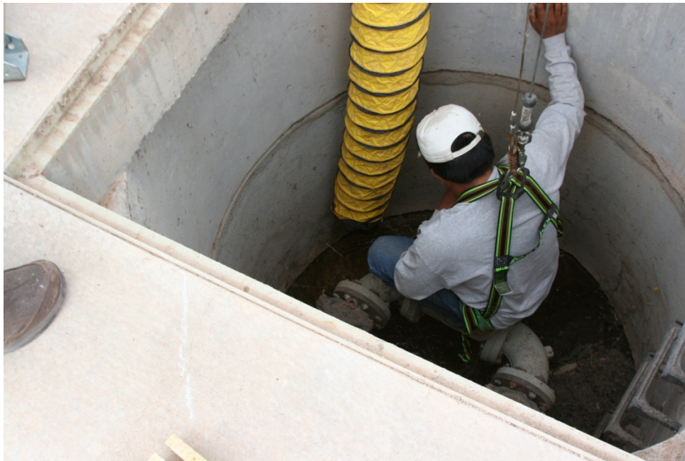
Entering a confined space with proper ventilation.
