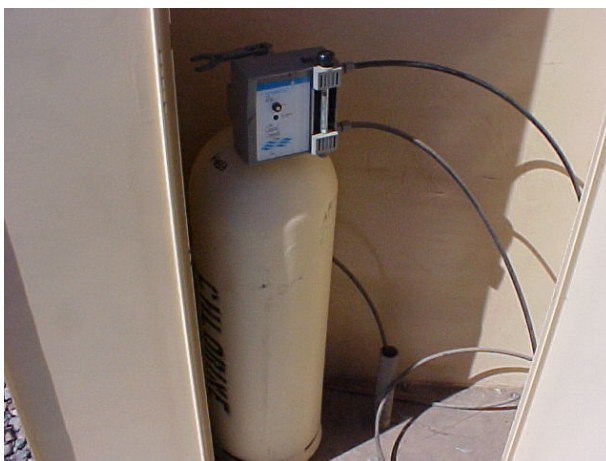
150 pound chlorine gas cylinder. Always tag the empty cylinder and store upright.
