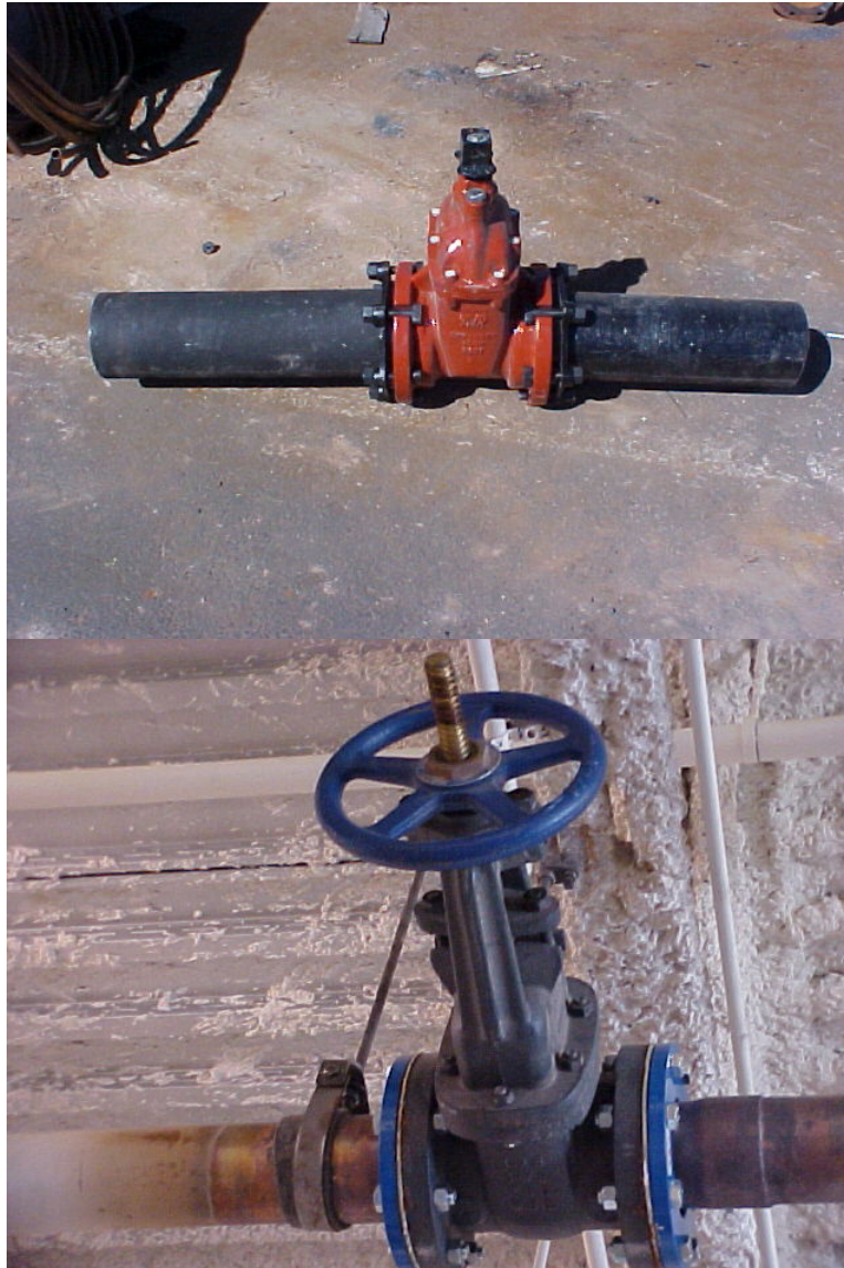
Two different styles of Gate Valves.
