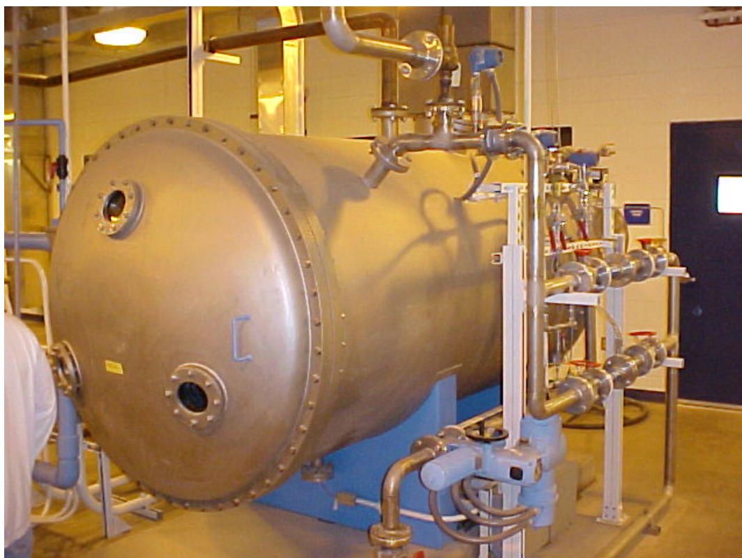
Ozone generator and Oxygen storage tank.
