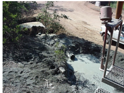
Constructed Mud Pits
