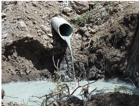
First Pit (heavy with cuttings)
