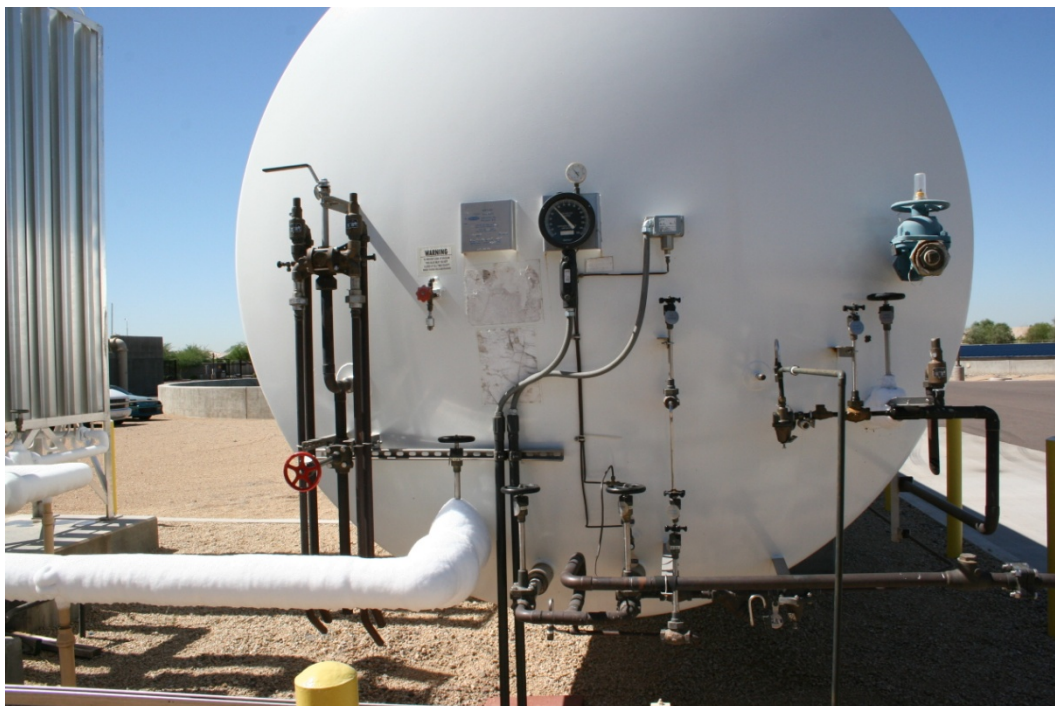
Ozone generator and Oxygen storage tank.
