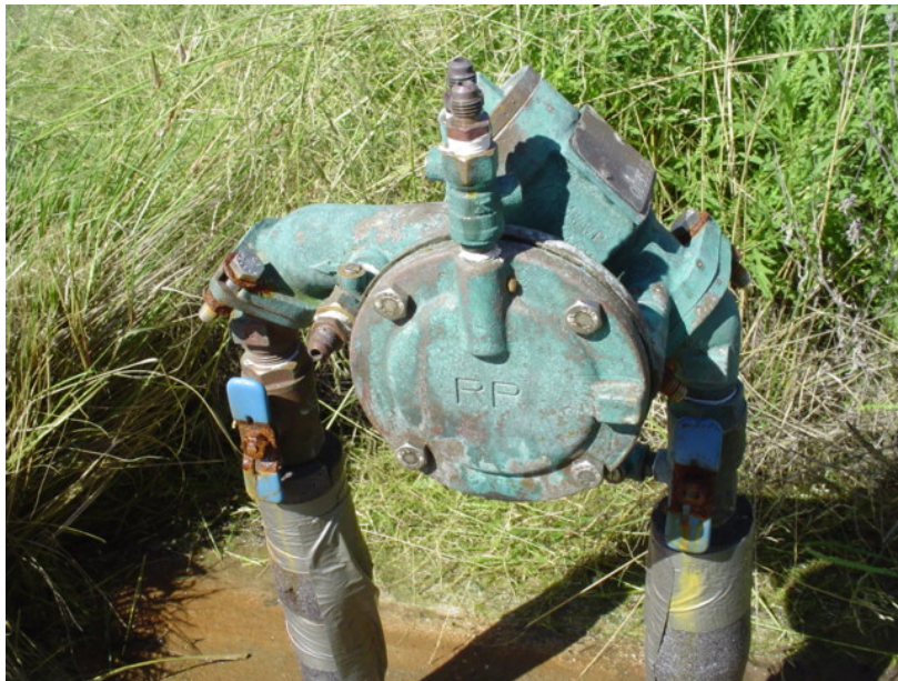
Various Reduced Pressure Principle Backflow Assemblies.
