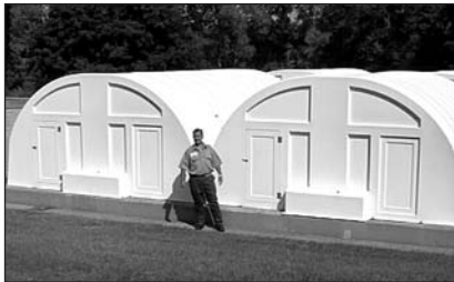
Above and at right: Rotating biological contactors (Secondary Treatment)
