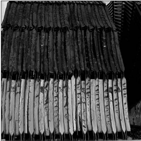
Above and at right: Rotating biological contactors (Secondary Treatment)
