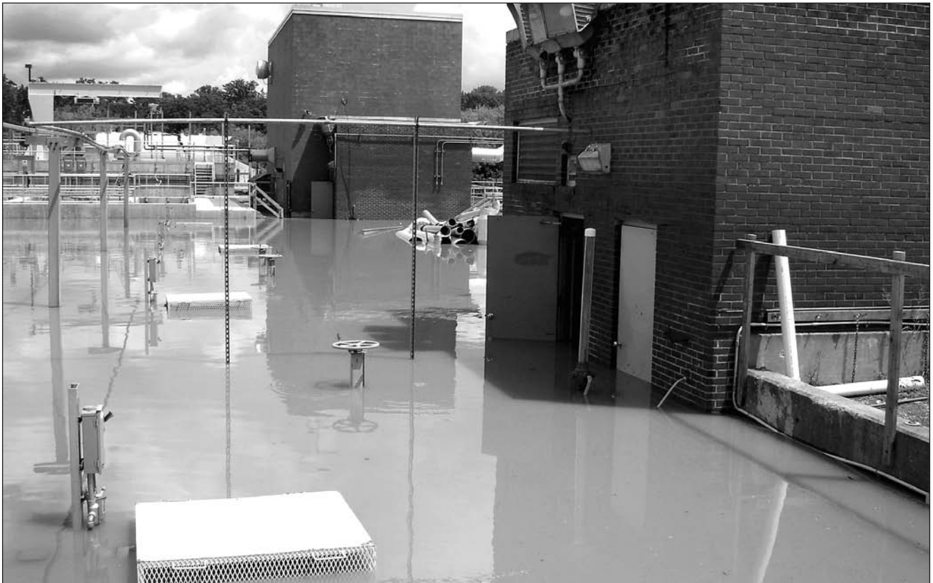
Binghamton-Johnson City Joint Sewage Treatment Plant (Summer 2006)
