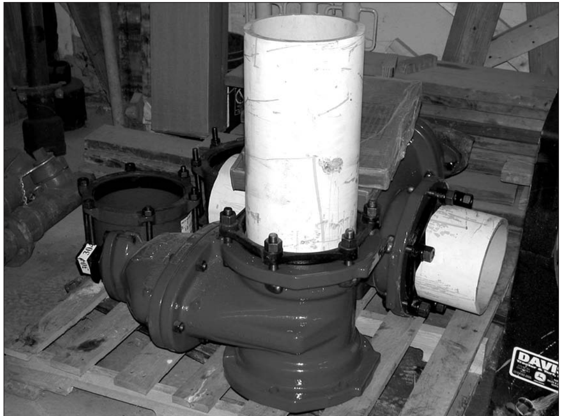
Replacement valve with preassembly awaiting installation
