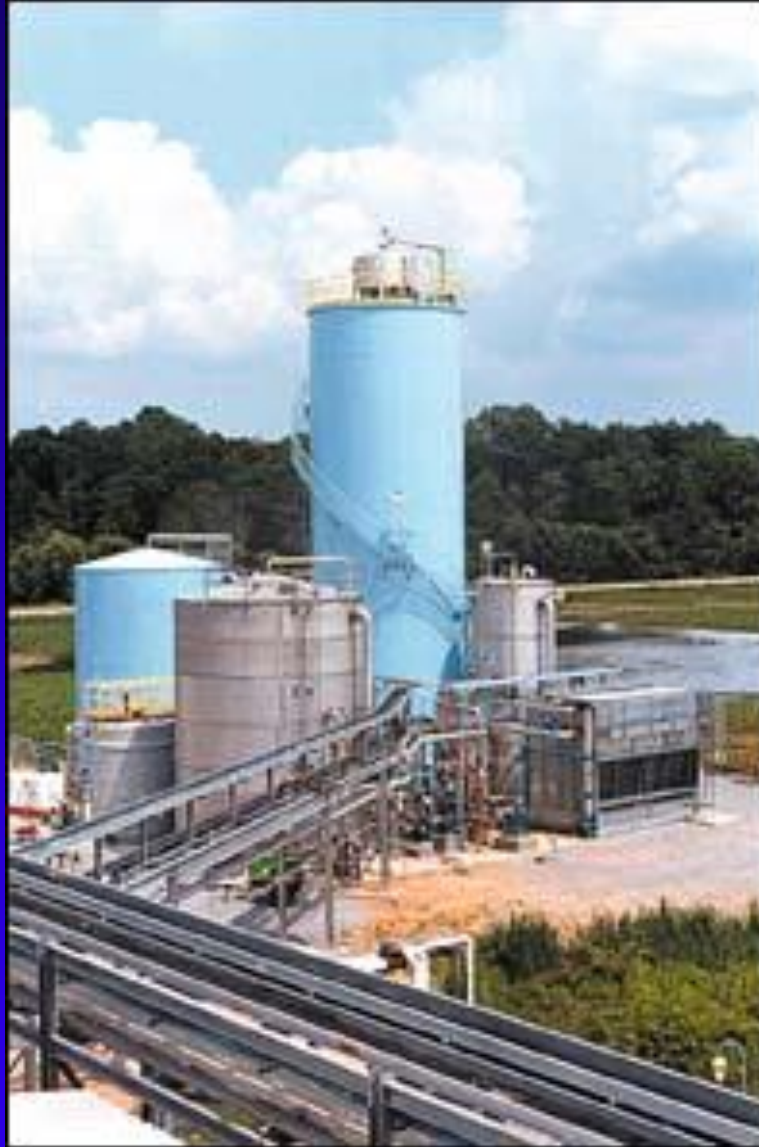
Kraft Paper Mill Foul Condensates, Alabama
