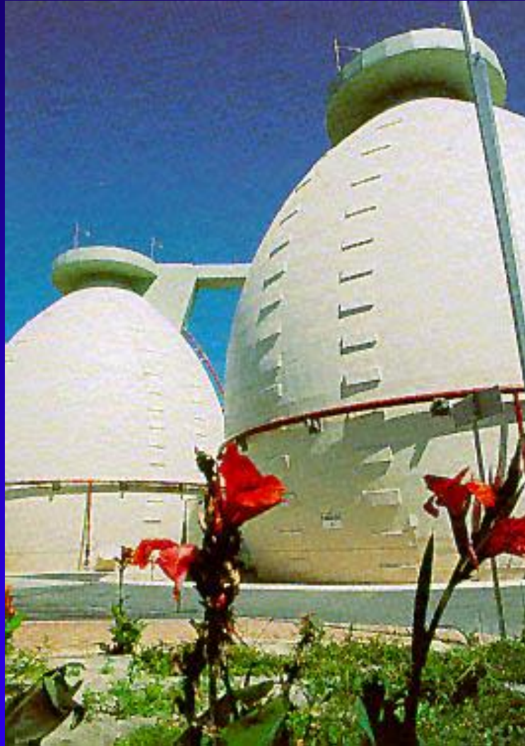
Municipal Sludge Digesters
