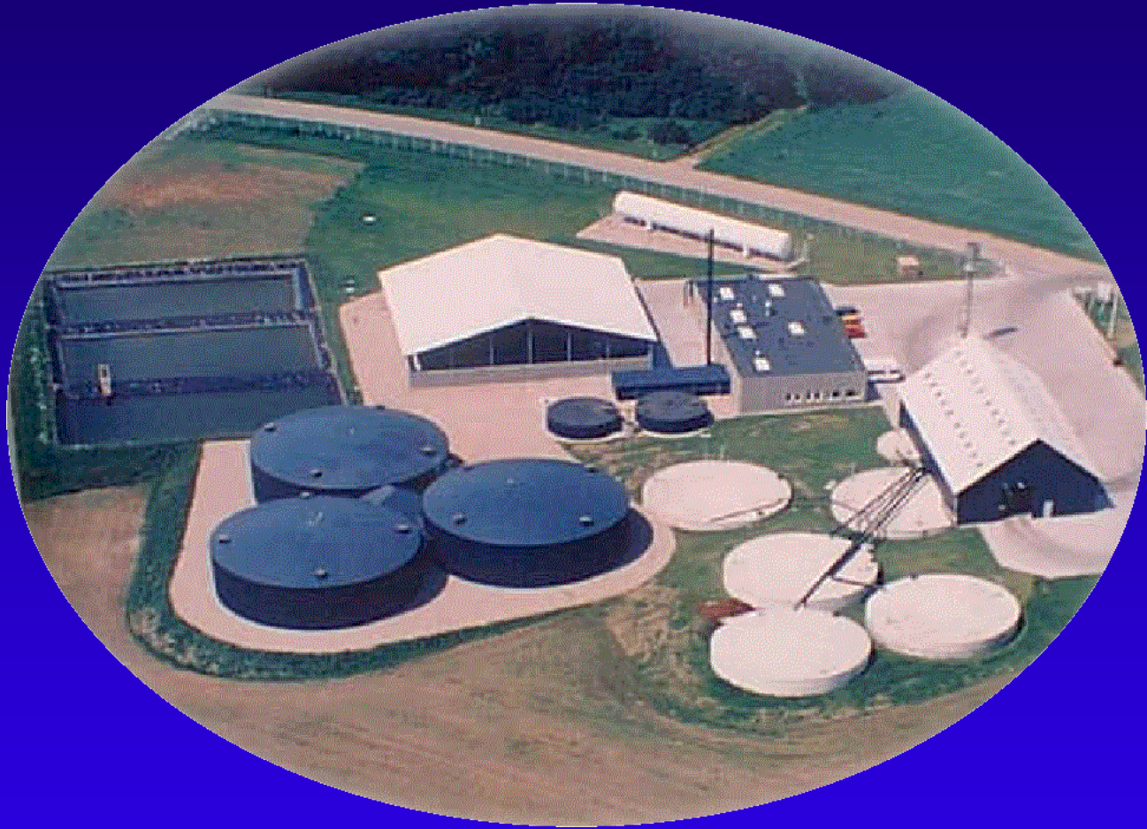
Lintrup Biogas plant (Denmark) animal manures
