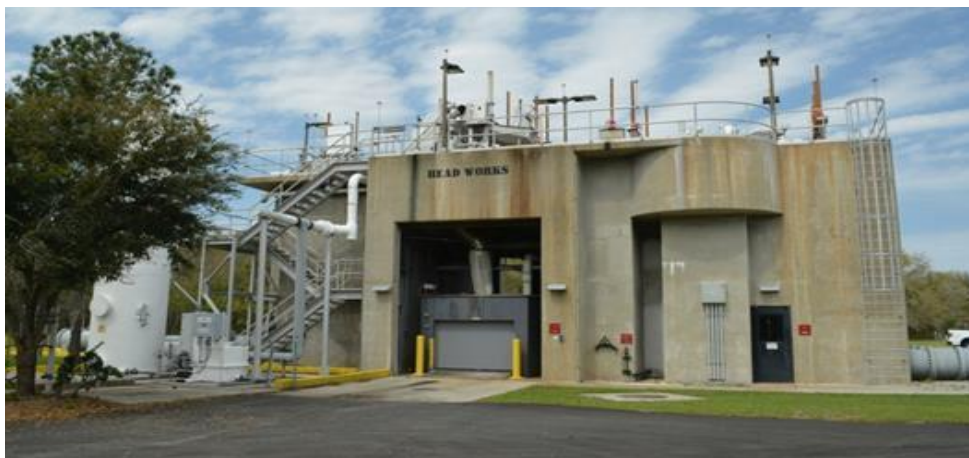
Figure 4-2 Primary Treatment (Headworks) at the Valrico Plant
