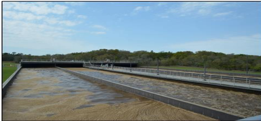
Figure 4-4 Secondary Treatment (Oxidation Ditch) at the Valrico Plant
