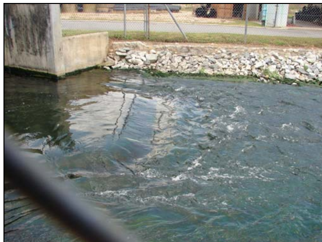
Figure 5. Beetham STP in Trinidad
