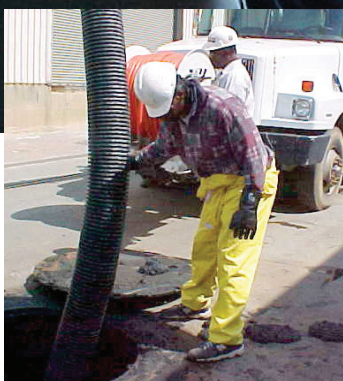
Sewer line maintenance
