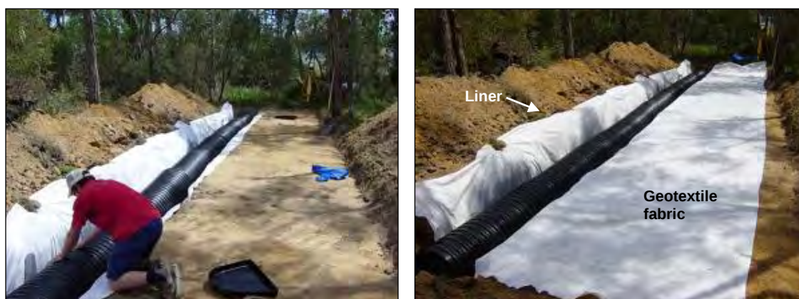
Figure 10.16 and 10.17 Laying the liner in the trench and then the geotextile fabric as the 'wick' across the pan
