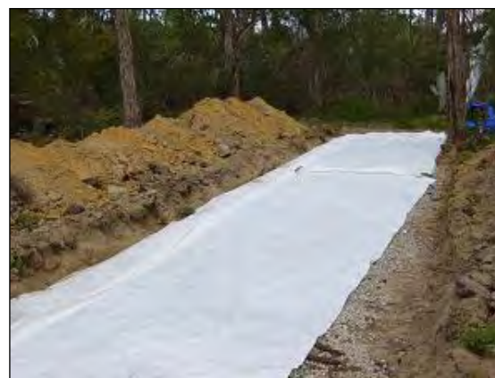
Figure 10.19 Adding the second geotextile fabric layer
