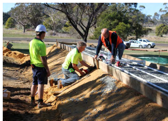
Figure 9.4 Constructing the manifold
