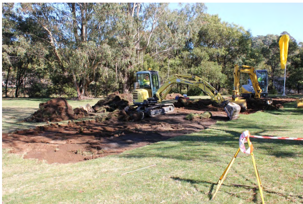
Figure 9.2 Excavation/preparation of base of mound
