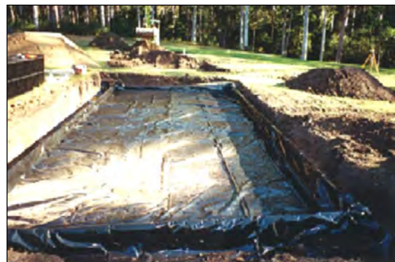
Figure 8.5 Lining with an impervious liner
