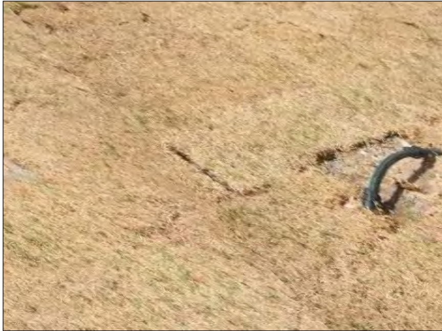
Figure 13.8 Damaged irrigation line sections cut out and replaced as part of an unsatisfactory repair.
