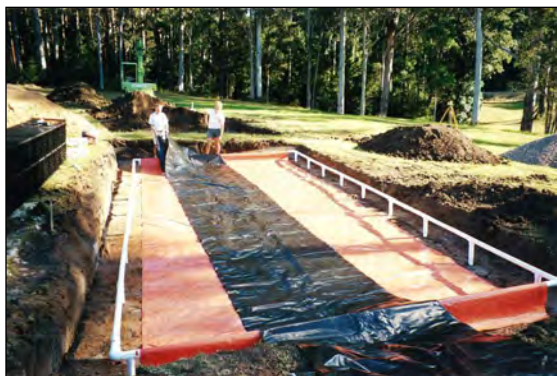
Figure 8.4 Construction membrane
