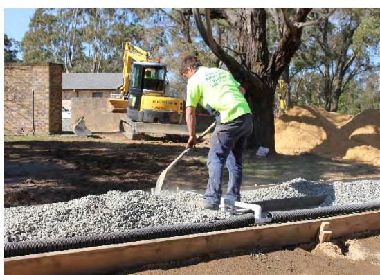
Figure 9.5 Gravel over inlet manifold
