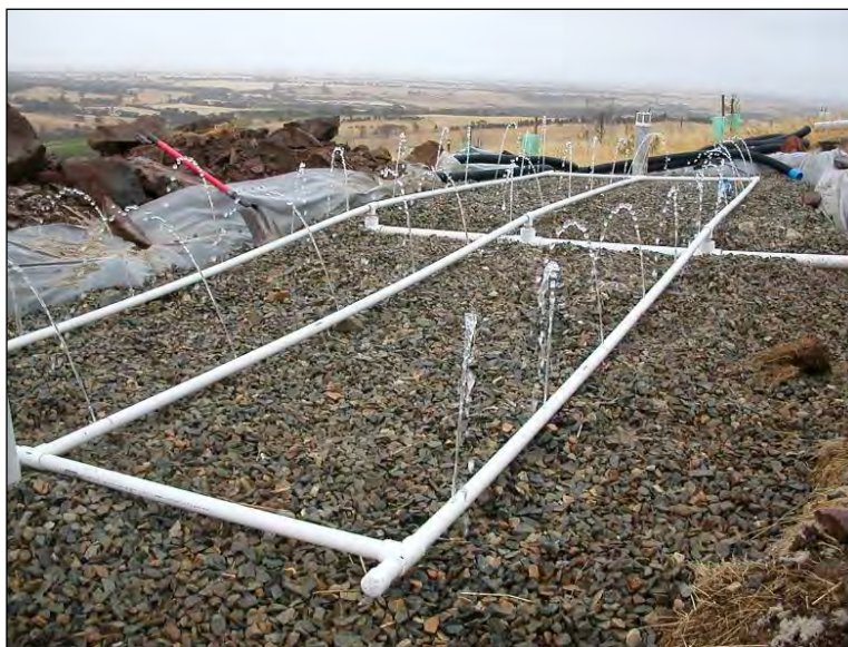
Figure 11.3 Pressure testing the distribution laterals for even distribution of effluent (Source: D Stafford)
