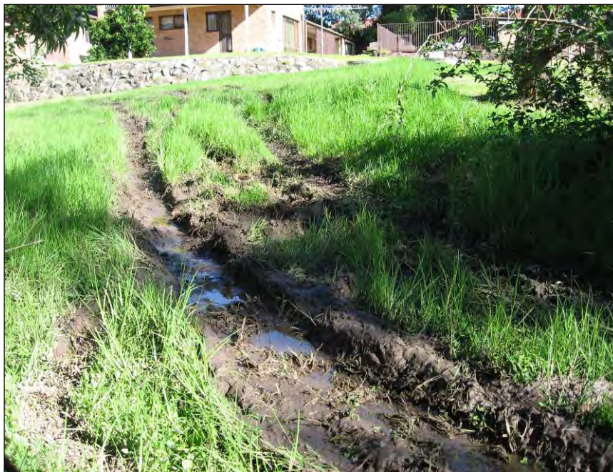
Figure 10.7 A failing trench due to vehicular activity
