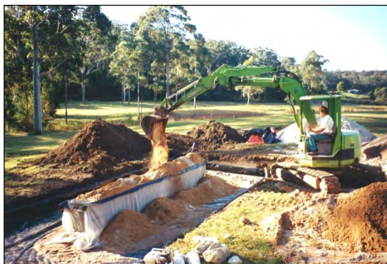
Figure 8.6 Backfilling with amended soil
