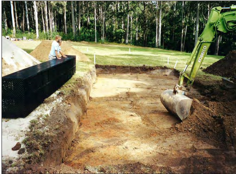
Figure 8.3 Excavation/preparation of base of mound (Figures 8.3-8.7 Ecomax, 2001)
