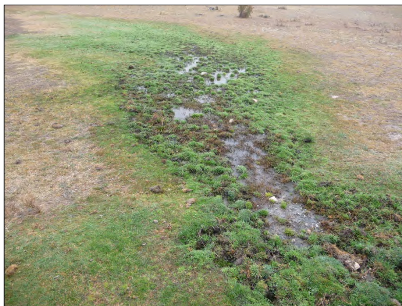
Figure 10.11 Failing trench
