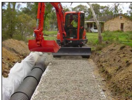
Figures 10.18 Backfilling gravel layer
