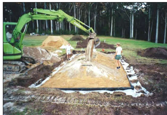
Figure 8.7 Final shaping of cell mound
