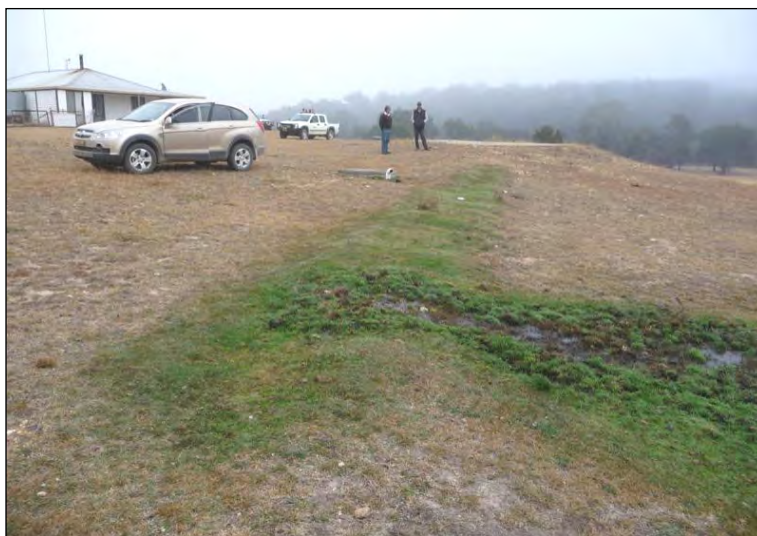
Figure 10.10 Failing trench
