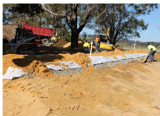
Figure 9.6 Sand on top of geotextile fabric
