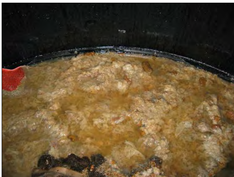
Figure 5.9 A flooded system due to pump failure
