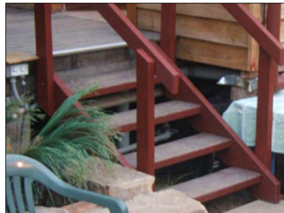
Figure 6.4 New steps blocking access to the composting unit
