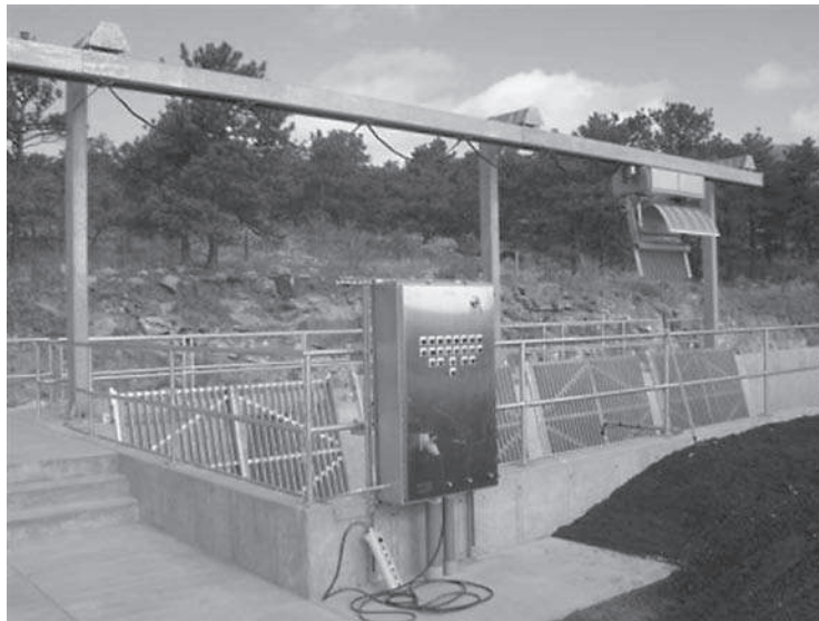
FIGURE 8.2 Coarse screen for onshore intake. (Source: Atlas.)
