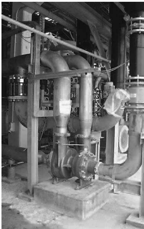
FIGURE 14.19 Turbocharger on 12,500 m 3 /day RO train.
