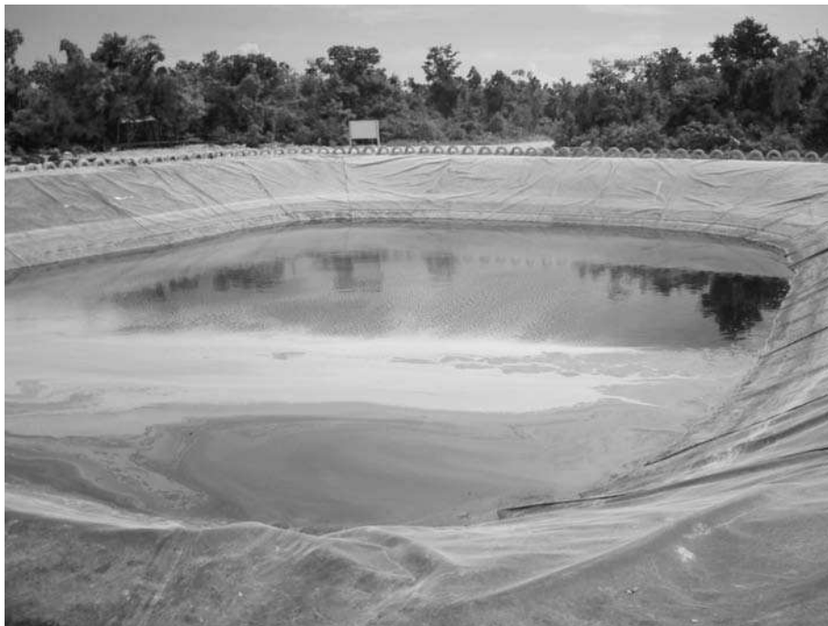
FIGURE 16.45 Geo-membrane evaporation pond liner.
