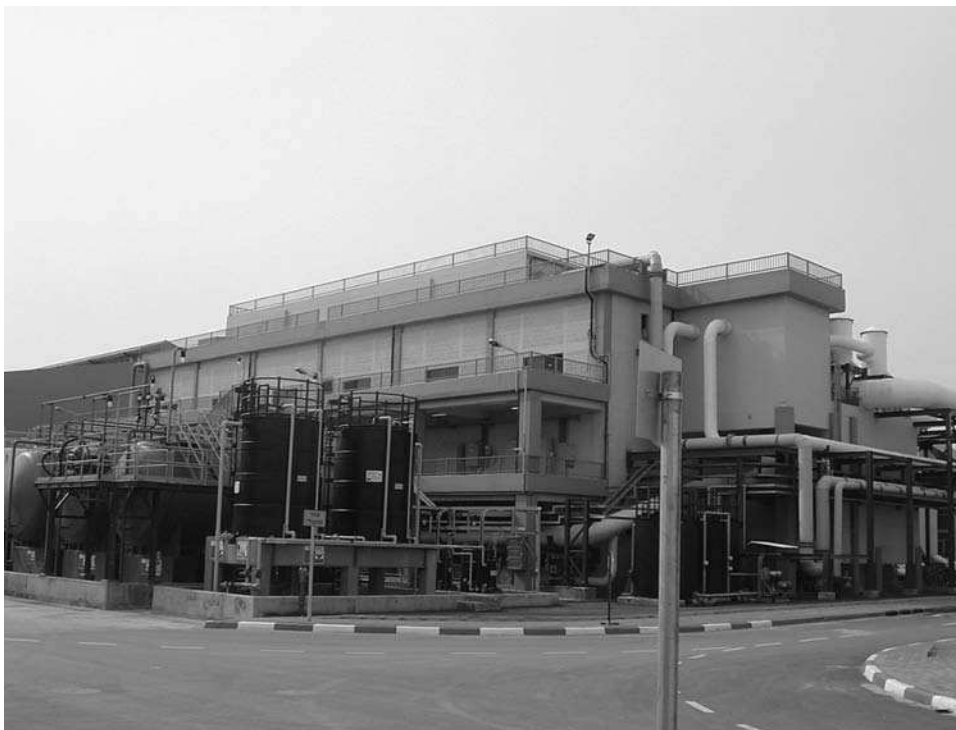
FIGURE 15.6 Calcite contactors of Ashkelon desalination plant, Israel.
