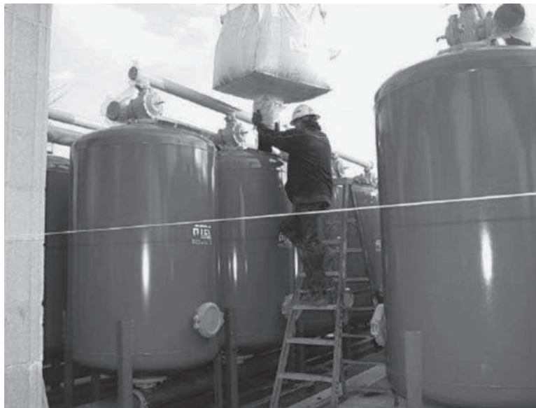
FIGURE 15.8 Refilling of calcite media.
