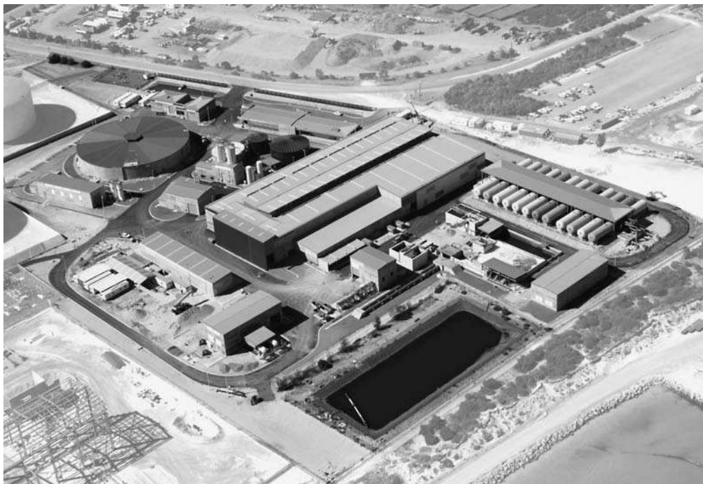
FIGURE 16.13 Perth seawater desalination plant. (Source: Water Corporation.)
