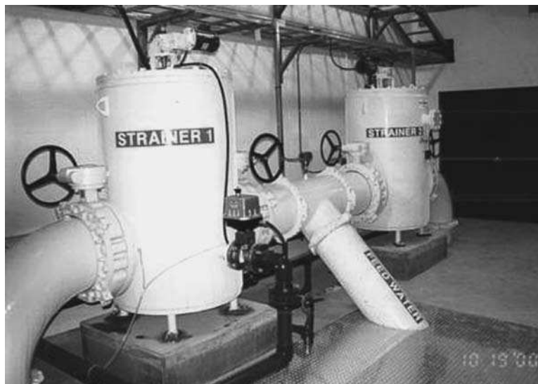
FIGURE 10.1 Sand strainers.
