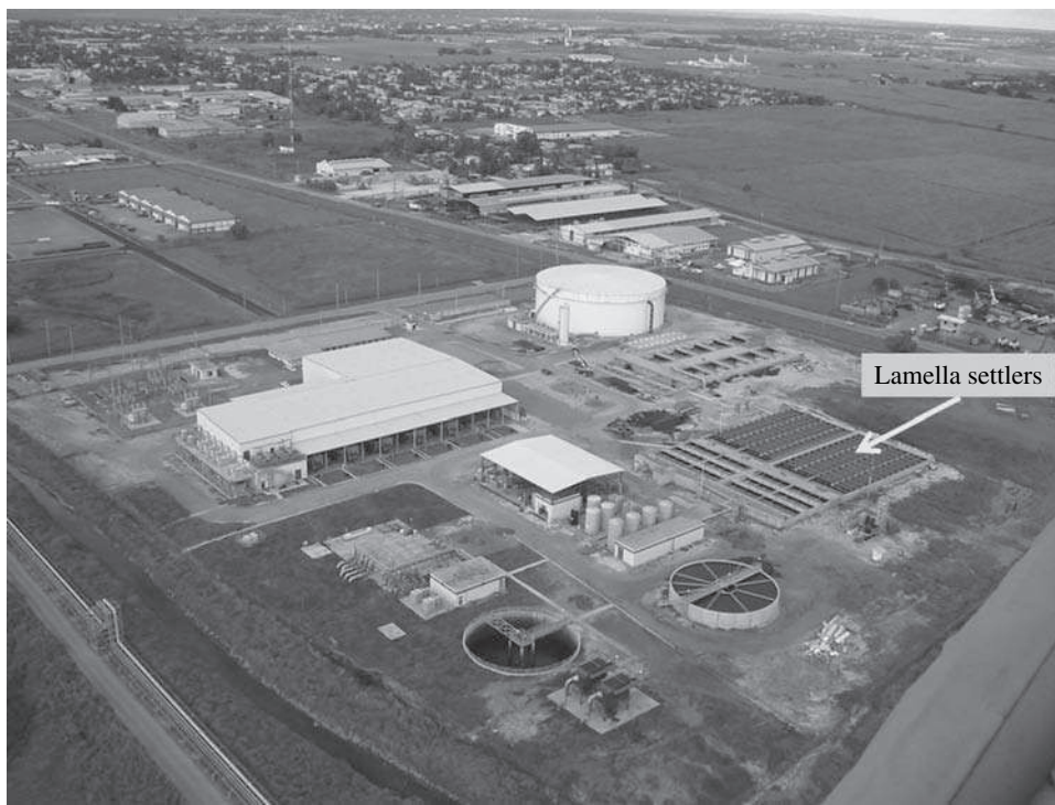
FIGURE 10.2 Point Lisas desalination plant, Trinidad. (Source: Desalcott.)
