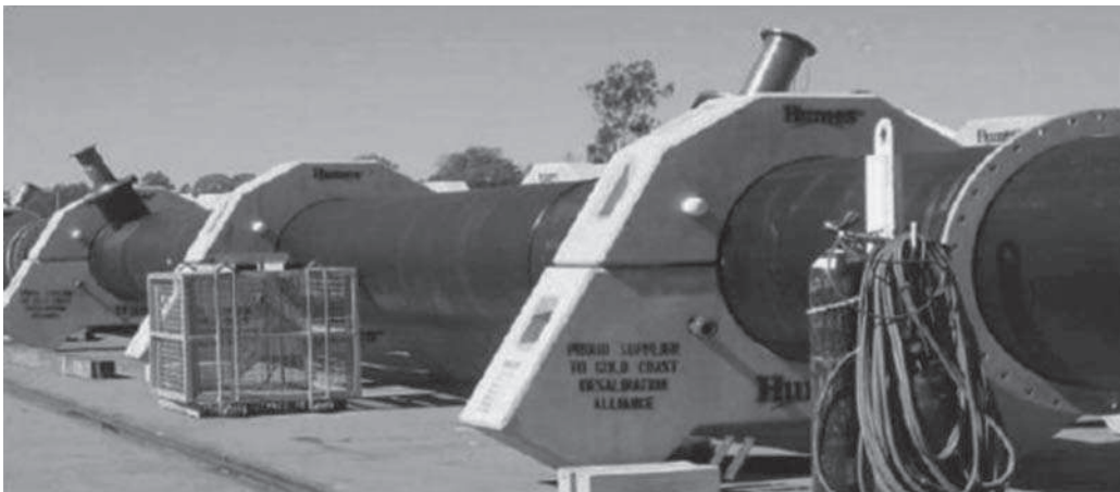
FIG.URE 16.7 Gold Coast SWRO plant diffuser.
