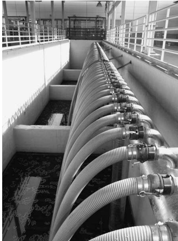
FIGURE 12.5 Submerged MF system.
