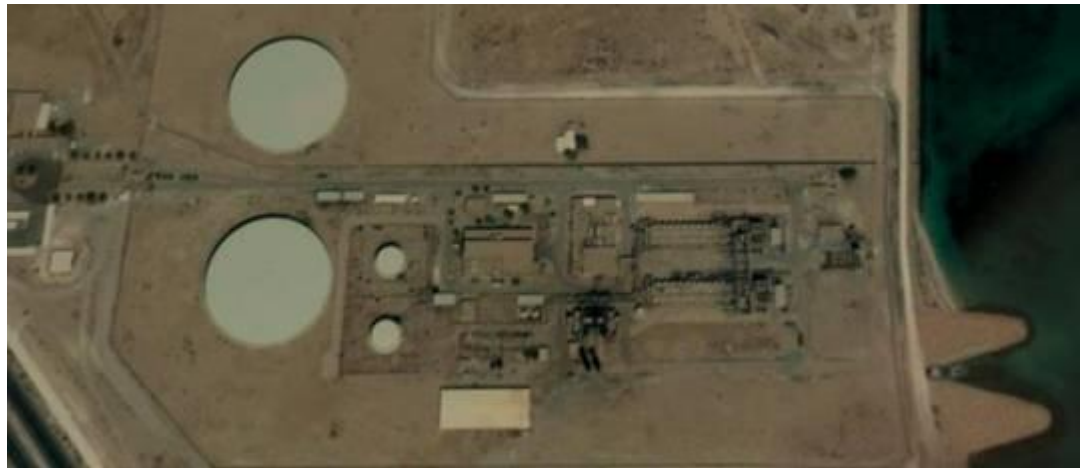
Existing Al Khafji plant
