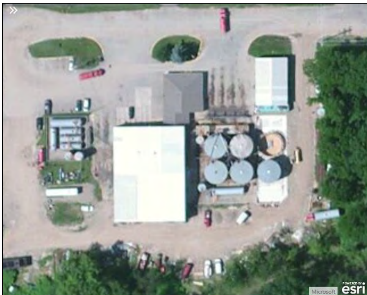
Figure 4-15. Aerial View of Waste Treatment Corporation Facility
