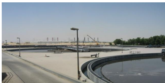
Secondary Sedimentation tank
