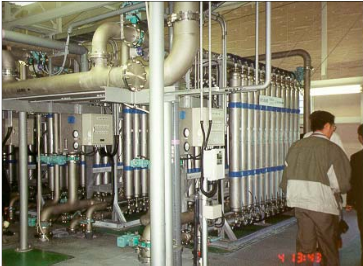
Membrane plant for water treatment, Ogoose Town, Japan
