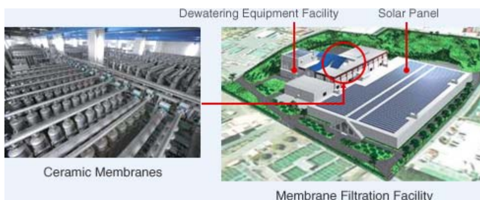
Figure 31: Envisaged Kawai Water Purification Plant under development by water next Yokohama Co.
