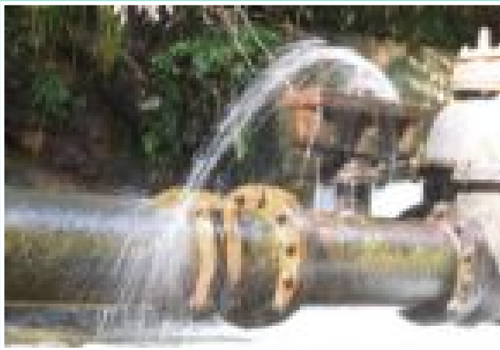
Leaking pipe
