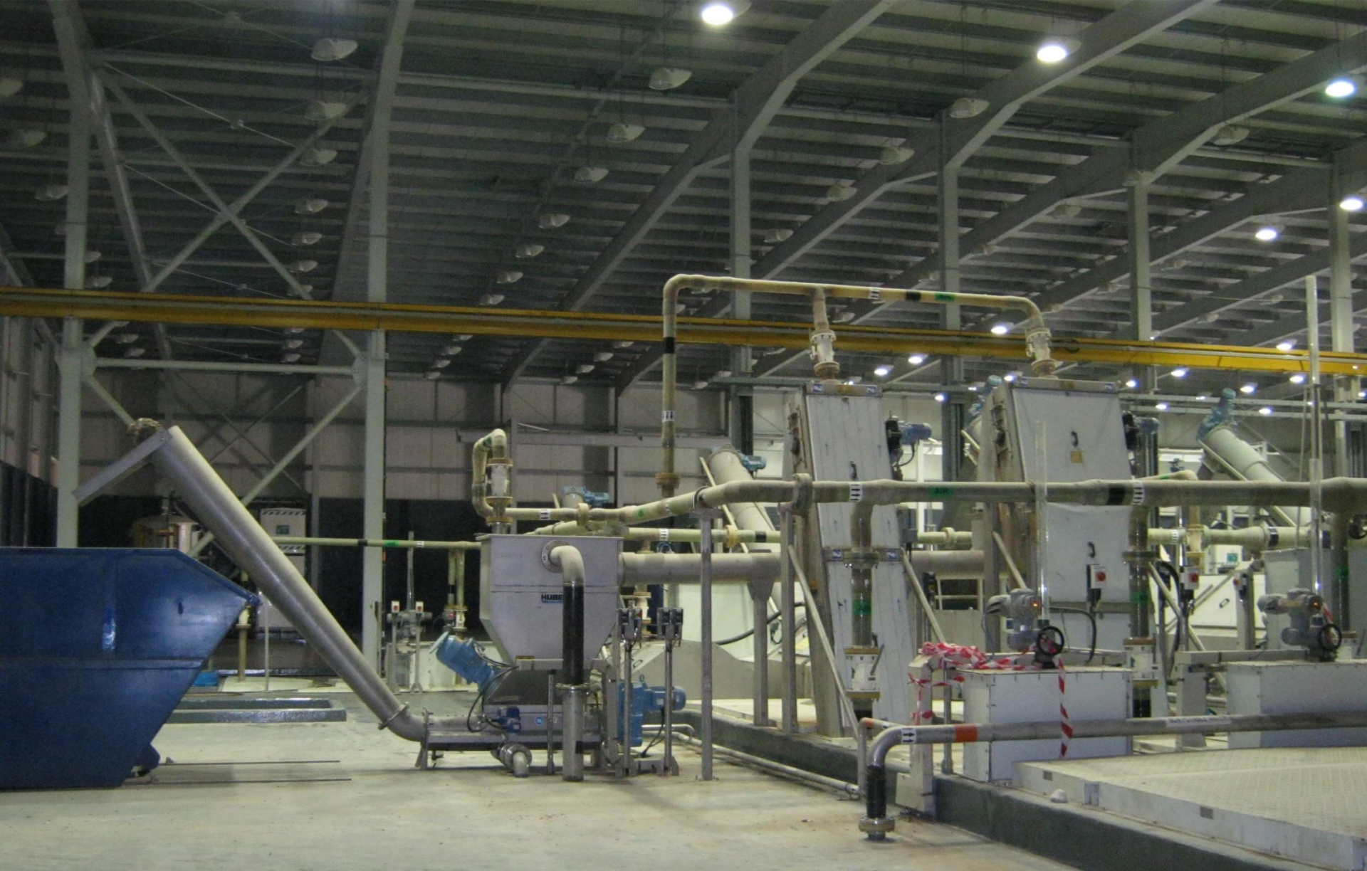
Screen Building (JASTP)
