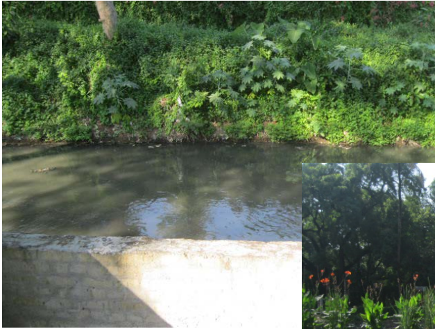
Raw sewage in nallah
