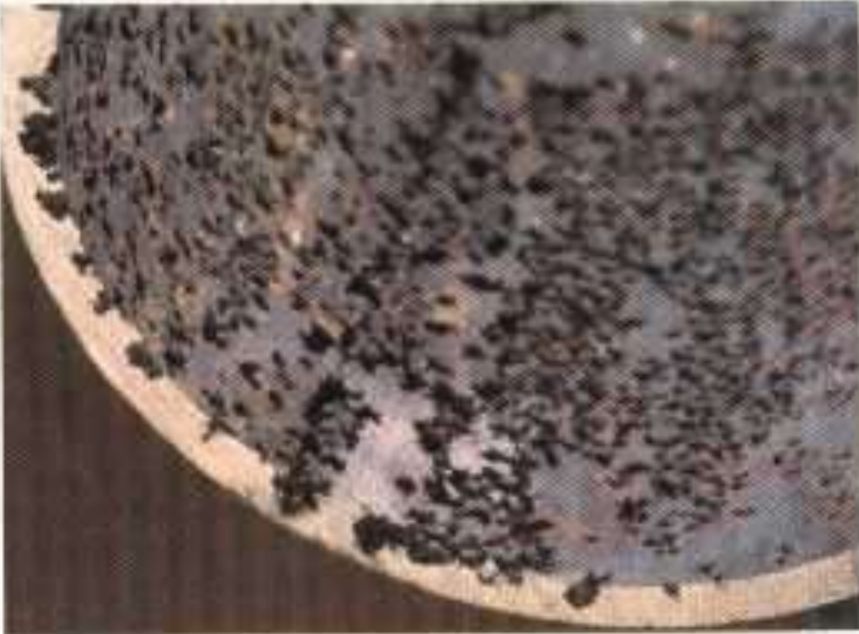
Oxygen pitting of a boiler feedwater pipe.
