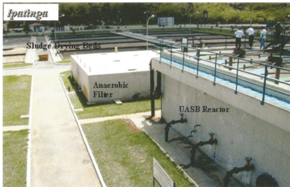
Figure 19: Photo of a UASB Reactor Followed by an Anaerobic Filter in Ipatinga, Minas Gerais, Brazil
