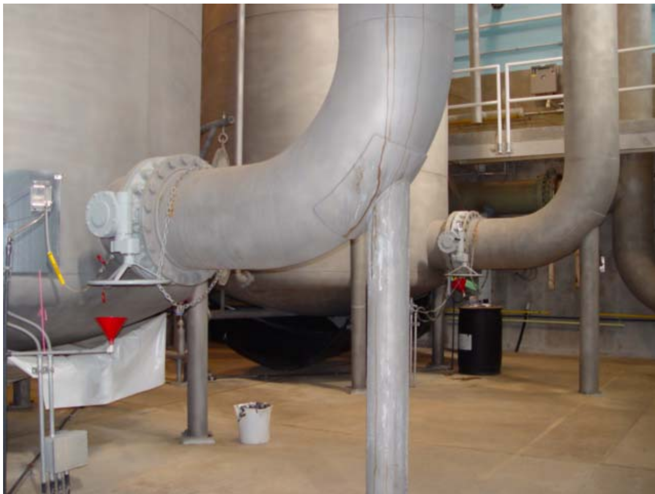
Figure 4.5 Stainless Steel Piping Showing Evidence of MIC Pinholes
