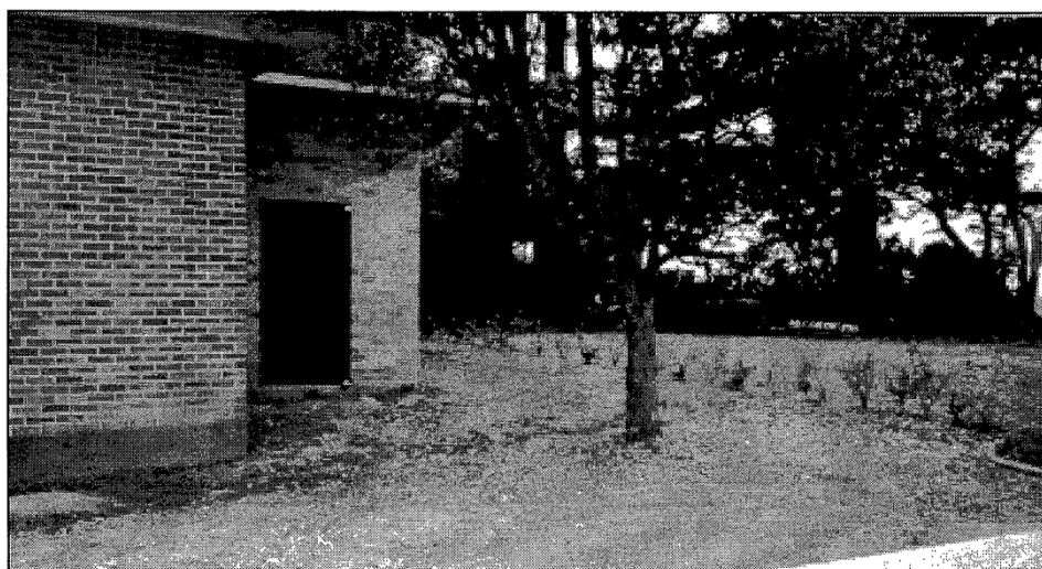
Mairangi Bay Pumping Station, with the new biofilter, soon after construction, shown to the right.
