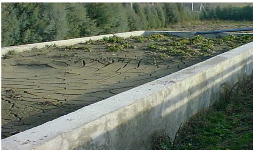
Figure 4. General view of drying beds.
