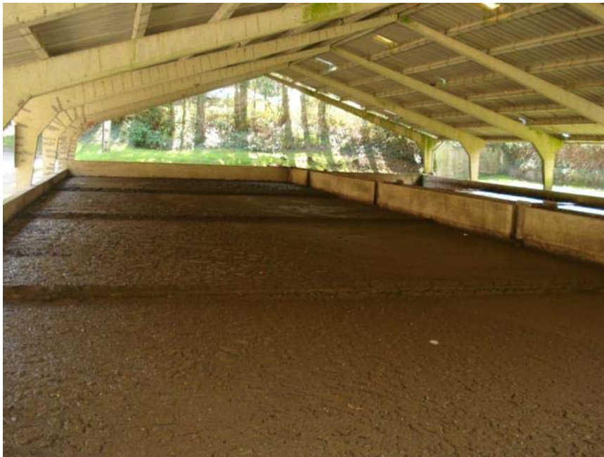
Figure 5. General view of a covered drying beds area.
