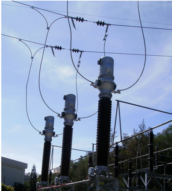
Figure 7: Potential Transformers
