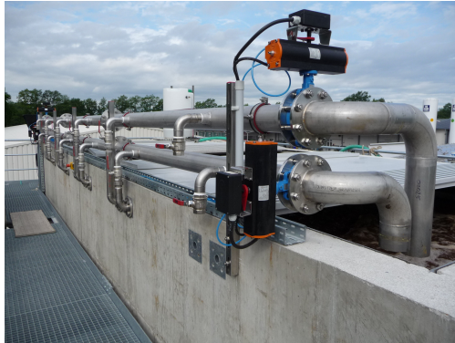
Scouring Air Manifolds
