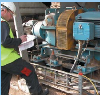
Mobile measurement, Diagnostic + troubleshooting service
