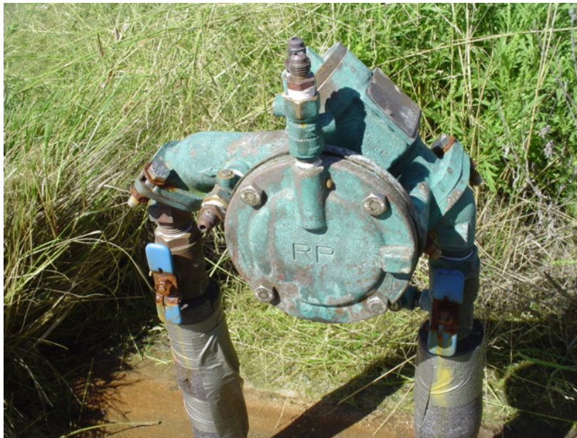
Various Reduced Pressure Principle Backflow Assemblies.
