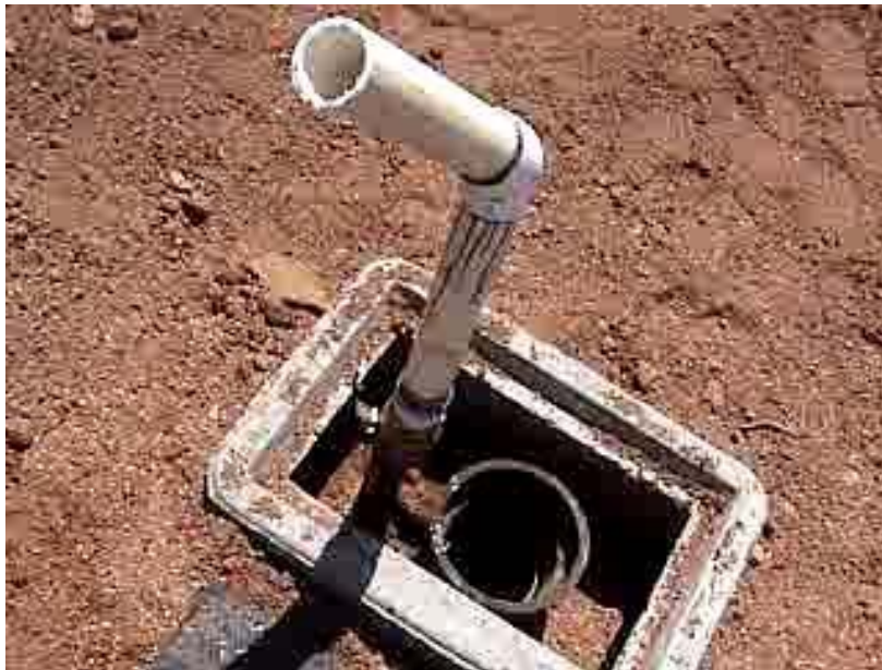
A temporary blow-off at a dead-end line.
