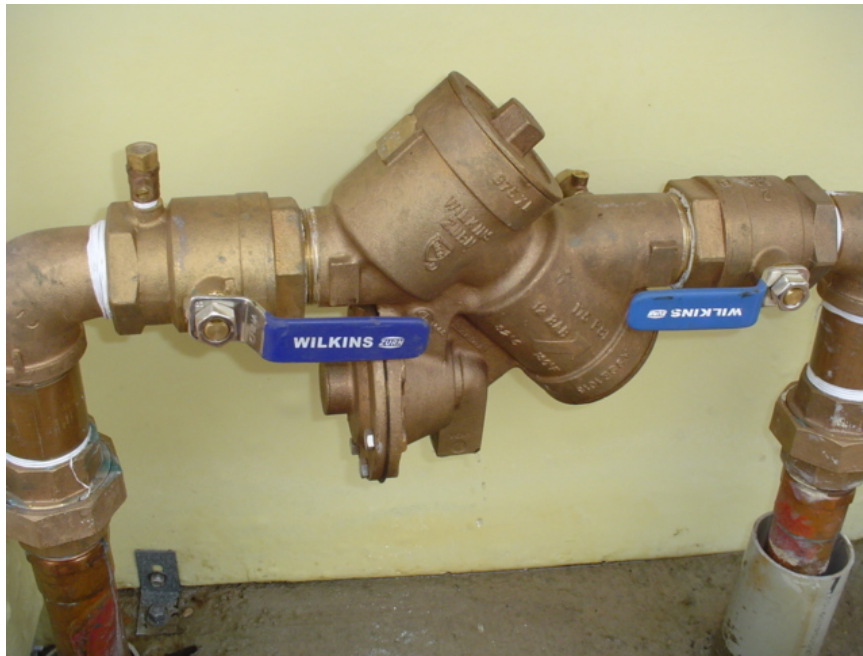
Various Reduced Pressure Principle Backflow Assemblies.
