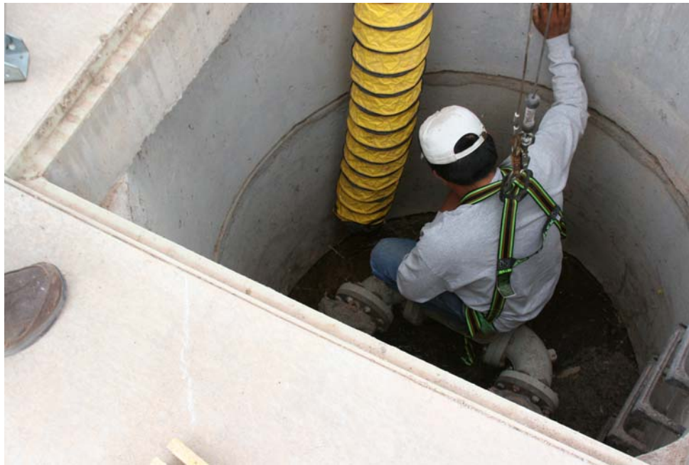
Entering a confined space with proper ventilation.
