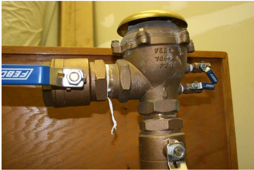
PRESSURE VACUUM BREAKER ASSEMBLY
