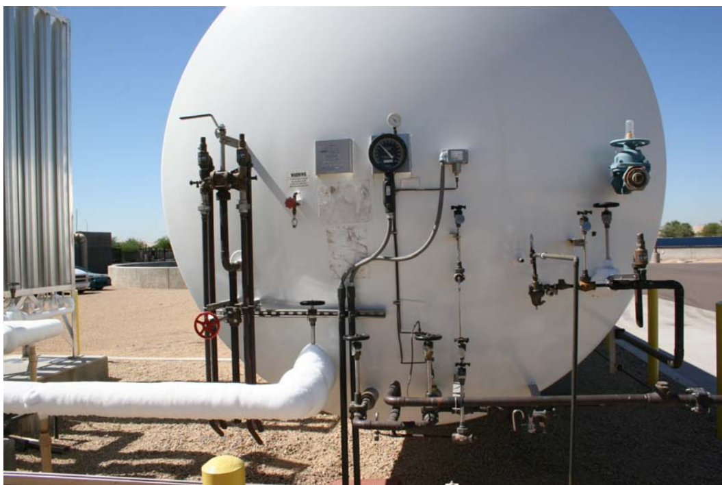
Ozone generator and Oxygen storage tank.
