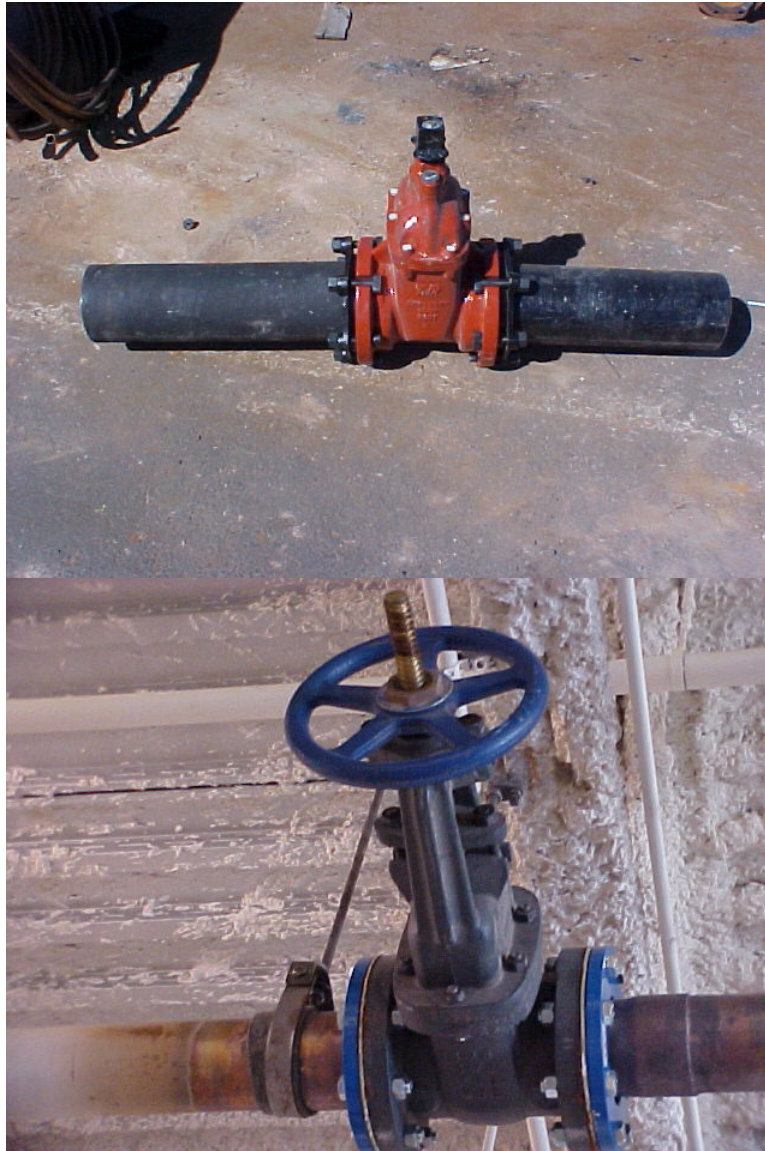
Two different styles of Gate Valves.
