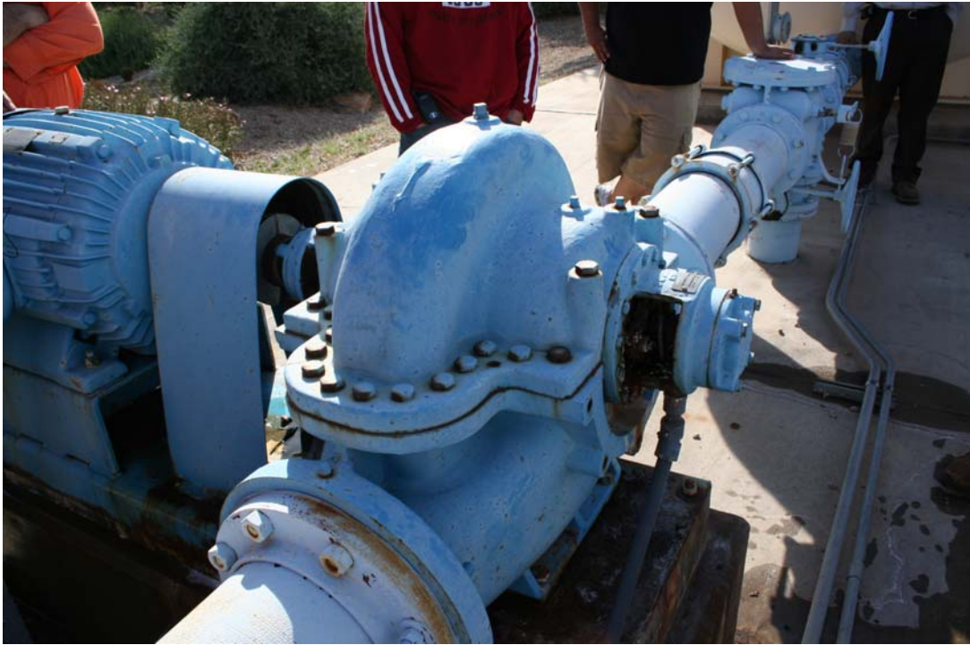
Split-case centrifugal pump.
