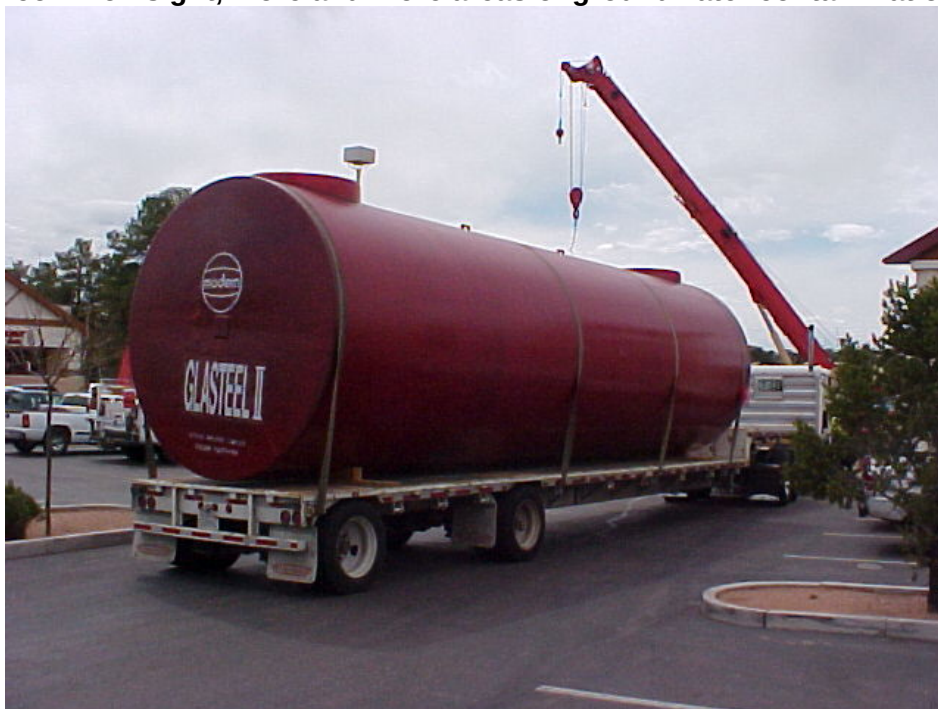
An underground Storage Tank, a source of pollution. L.U.S.T.
