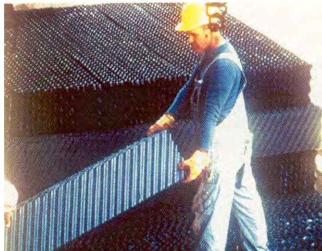
Figure 4-11. High-Efficiency Cooling Tower Film Fill
