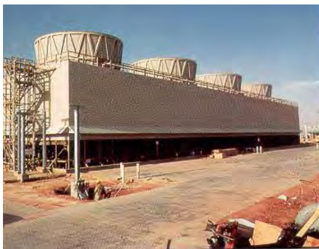
Figure 4-9. Counter-Flow Cooling Tower
