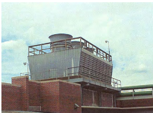
Figure 4-7. Cross-Flow Cooling Tower
